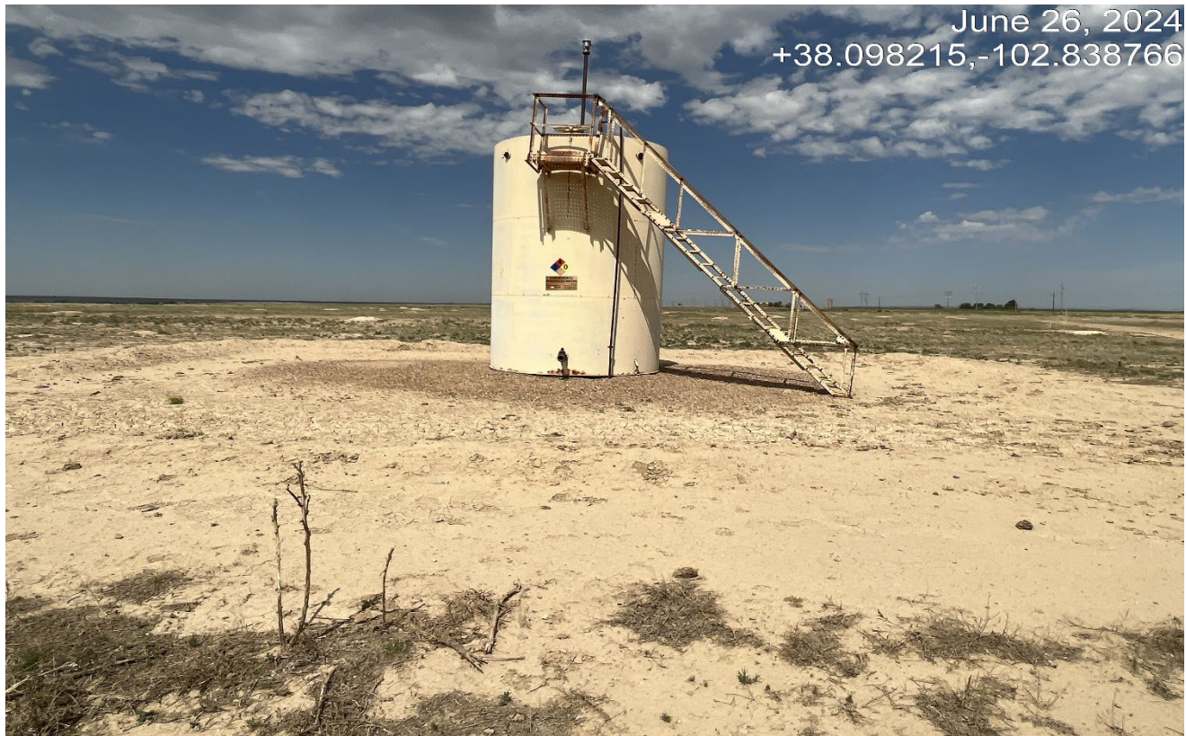
Photo 2. Facing toward the tank battery. There is insufficient secondary containment to contain a spill. Previous CA was not completed.
