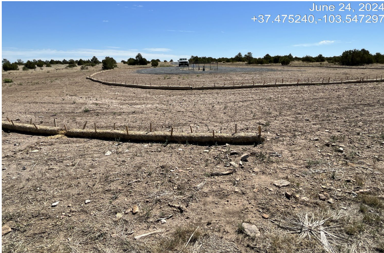
Photo 6. Facing east at the location. The straw wattles have been placed at the disturbance area and where the slope is at the northwest side of location.
