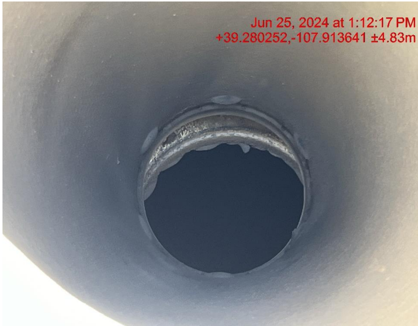
Thief hatch open to wildlife/atmosphere - Photo #03007
