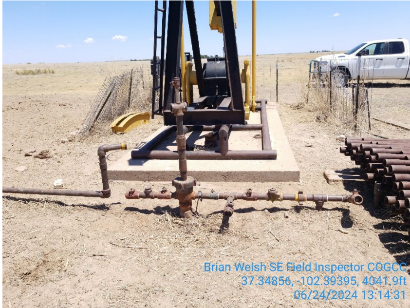
Wellhead and water leg
