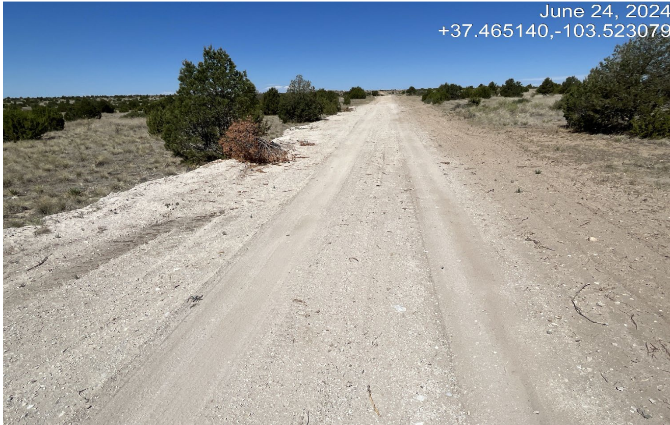
Photo 10. Facing west along the flowline. The vegetation is not establishing and soils are whitish and don't match the surrounding soils. Topsoil was not salvaged along the flowline which could be impacting revegetation. There are also vehicle tracks along the flowline causing unnecessary disturbance.
