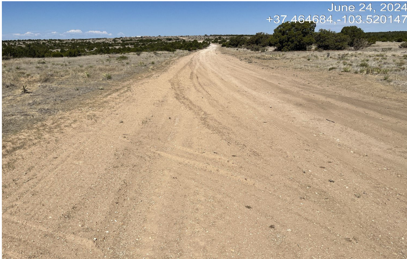
Photo 2. Facing back west toward the flowline disturbance. The vegetation is not establishing along the flowline and there are vehicle tracks which a causing unnecessary disturbance. The flowline must be reclaimed and stabilized.
