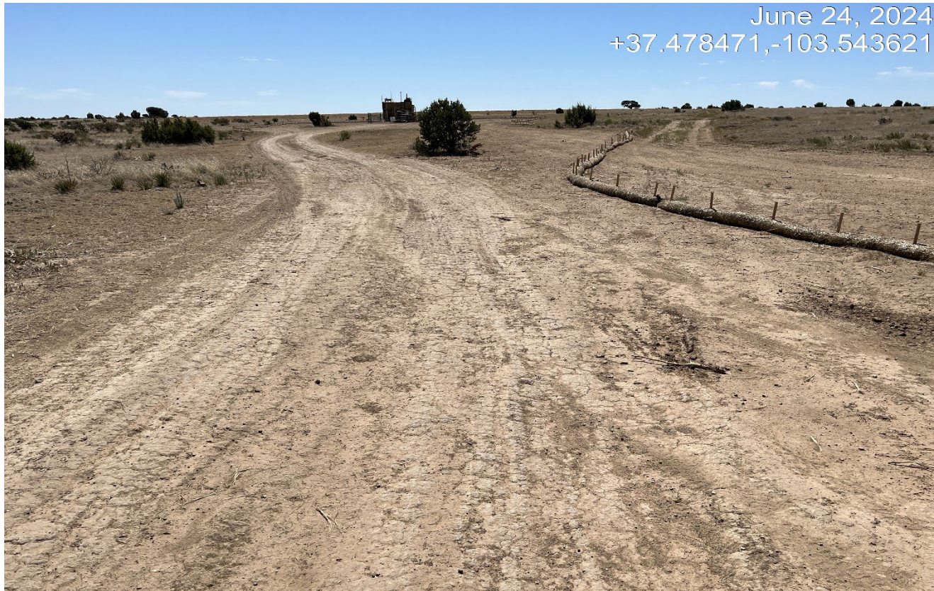
Photo 1. Facing east toward along the access road near the location. Topsoil was not salvaged along the road and soils are very compacted.
