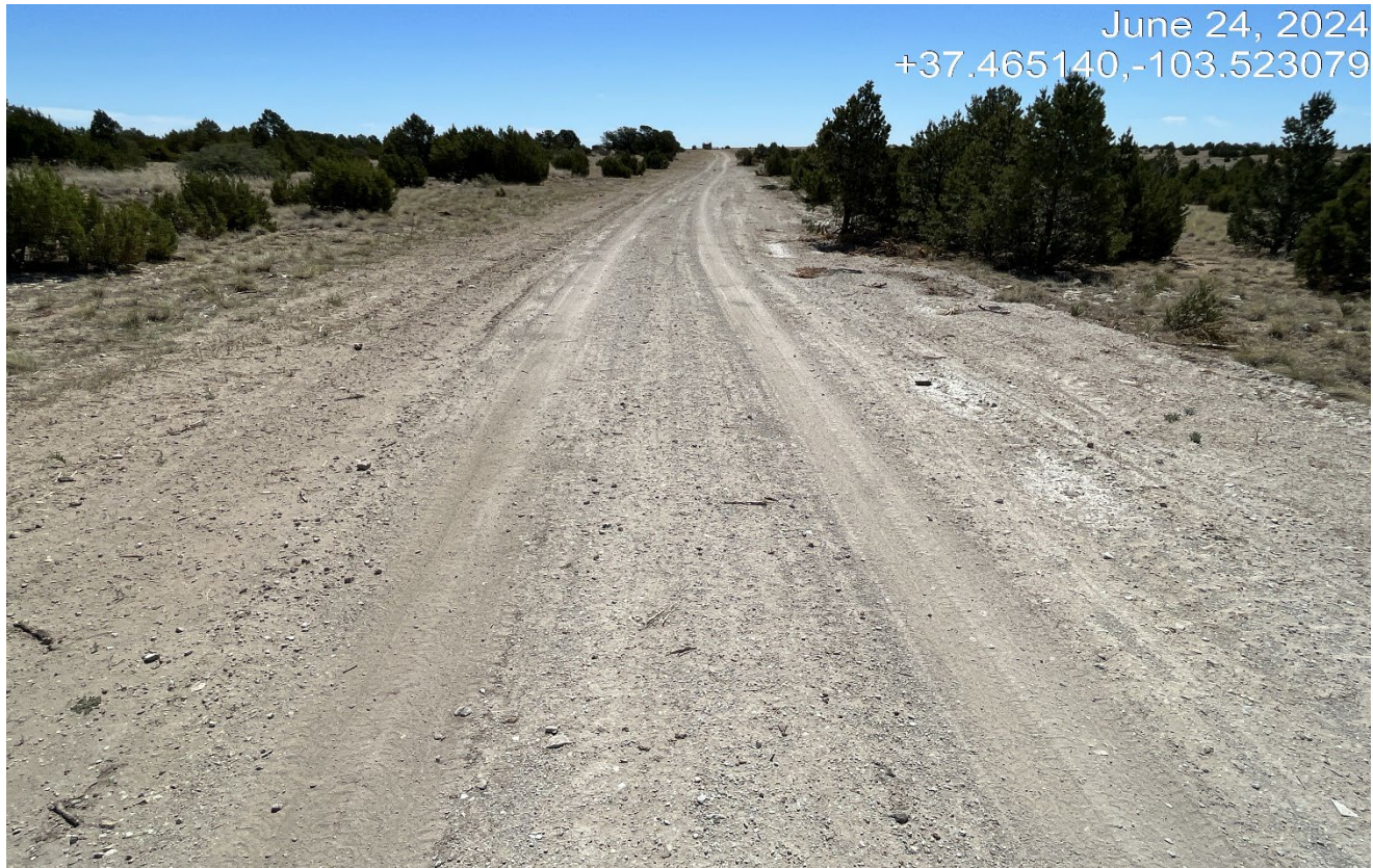
Photo 9. Facing east along the flowline. The vegetation is not establishing and soils are whitish and don't match the surrounding soils. Topsoil was not salvaged along the flowline which could be affecting vegetation. There are also vehicle tracks along the flowline causing unnecessary disturbance.
