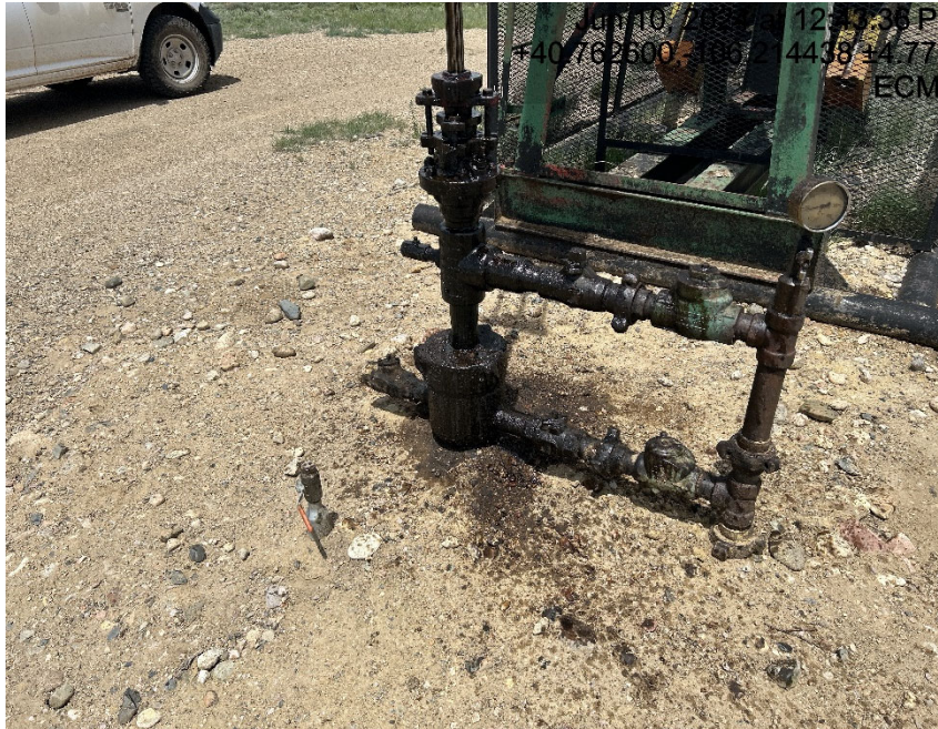
Well head leaking
