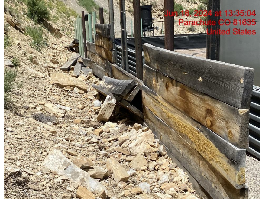
Insufficient Erosion Control/Degradation/Debris – Photo #01785
