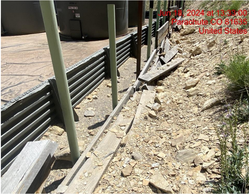
Insufficient Erosion Control/Degradation/Debris – Photo #01781
