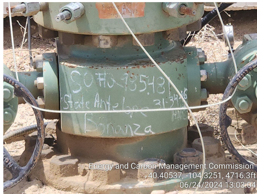
Photo 8 – Wellhead Sign missing
