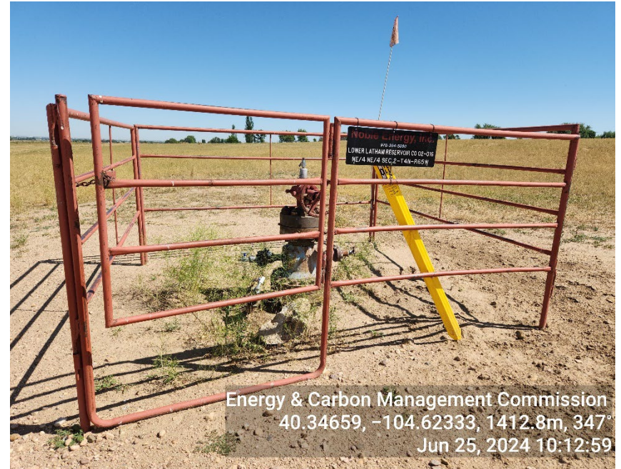
Photo 2: TA wellhead, overgrown vegetation
