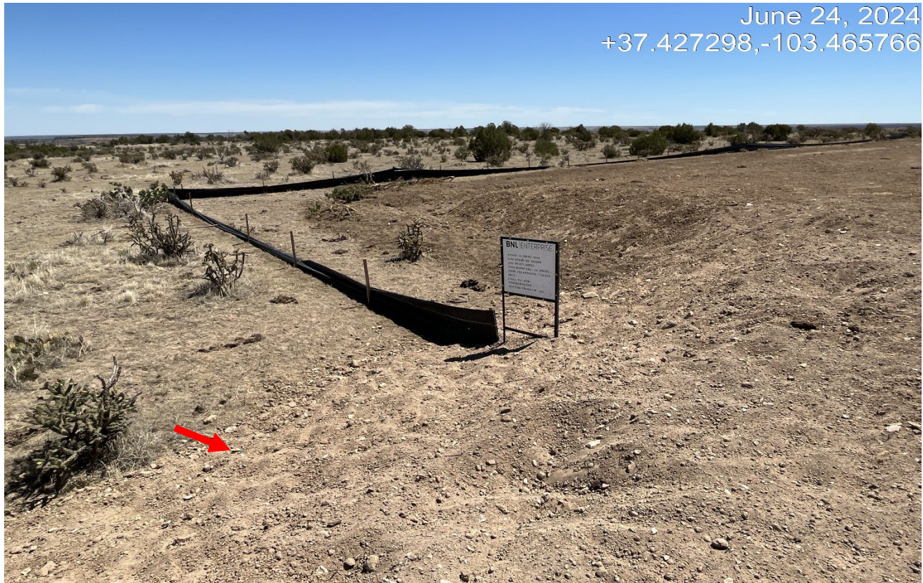
Photo 2. Facing toward the northwest side of the location. The silt fence is not maintained at the location. The loose soils along the access road at red arrow are not stabilized.
