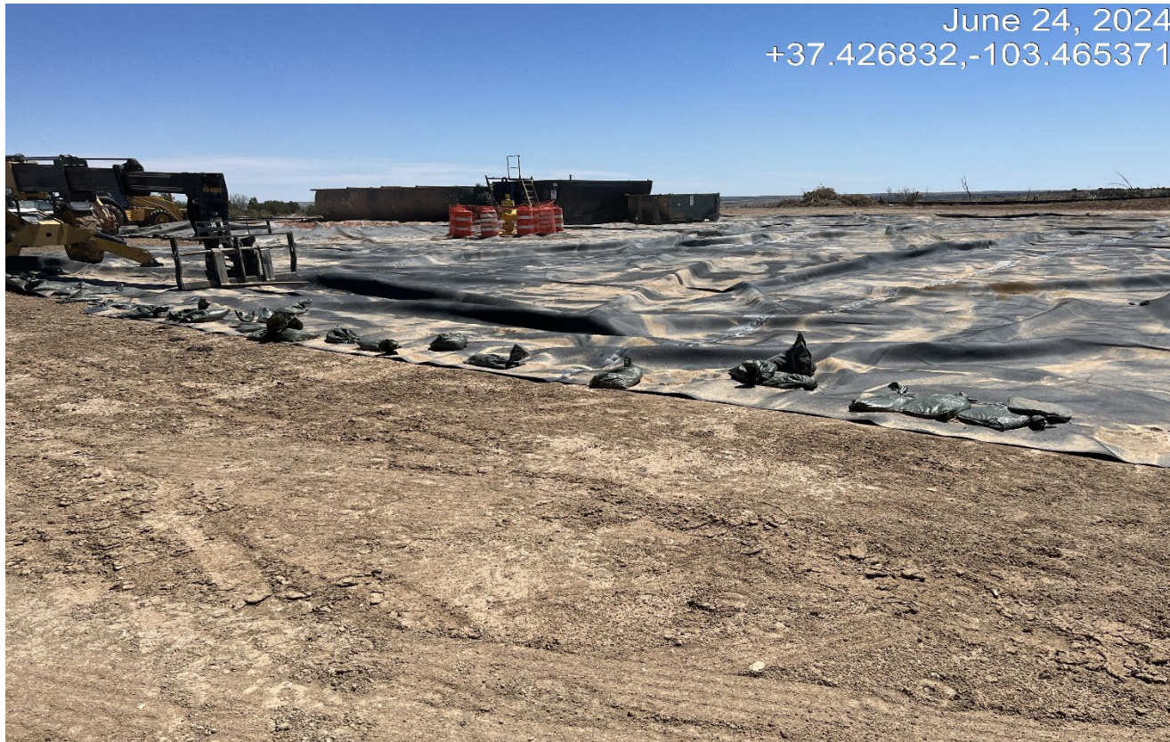
Photo 3. Facing northeast at the location. The well has been drilled and liner was used during the drilling process..
