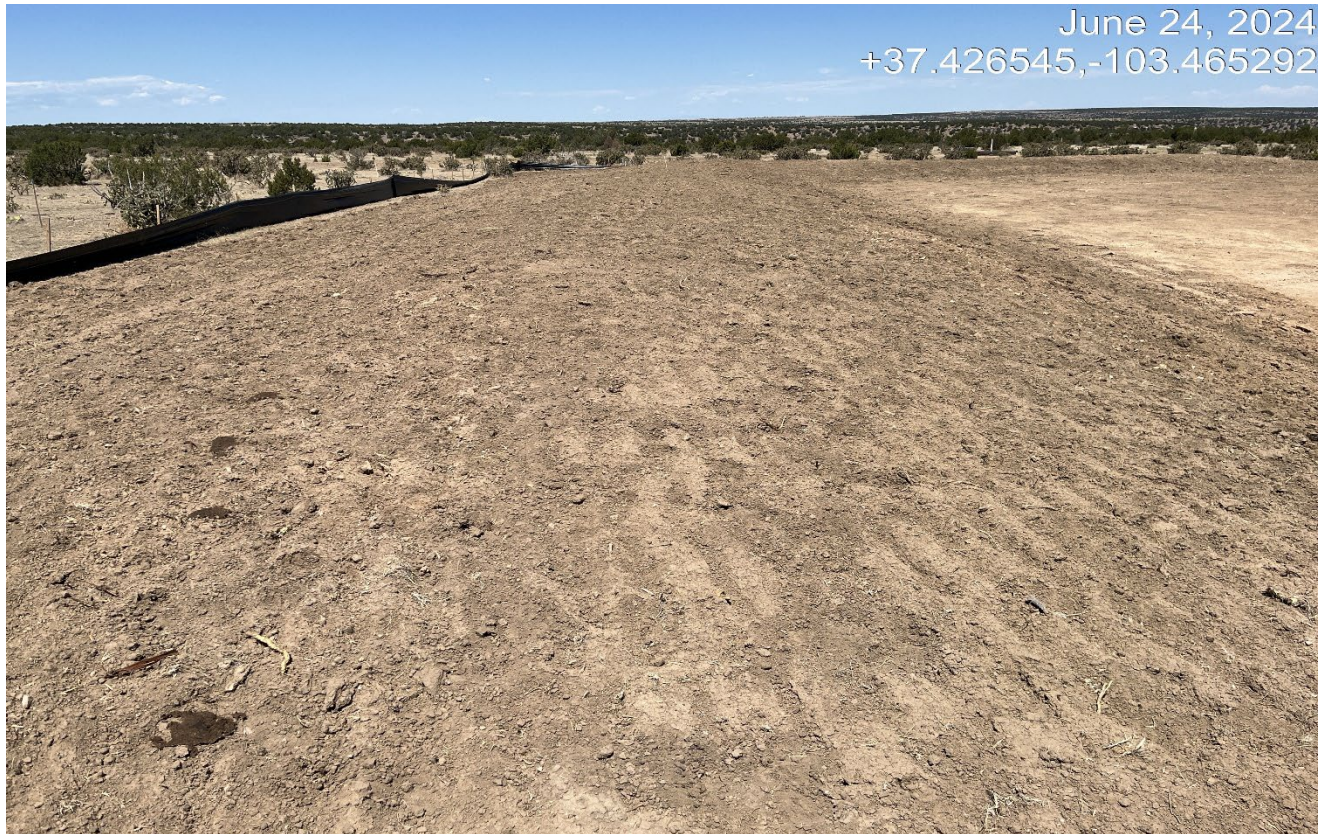
Photo 8. South side of the location facing west toward the topsoil pile. The topsoil has not been seeded and is not stabilized.
