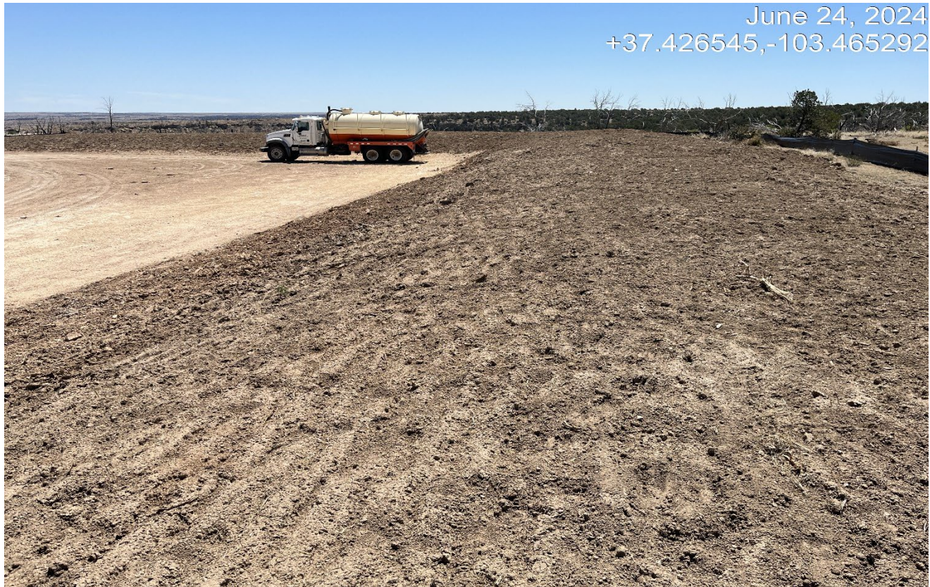
Photo 7. South side of the location facing east toward the topsoil pile. The topsoil has not been seeded and is not stabilized.
