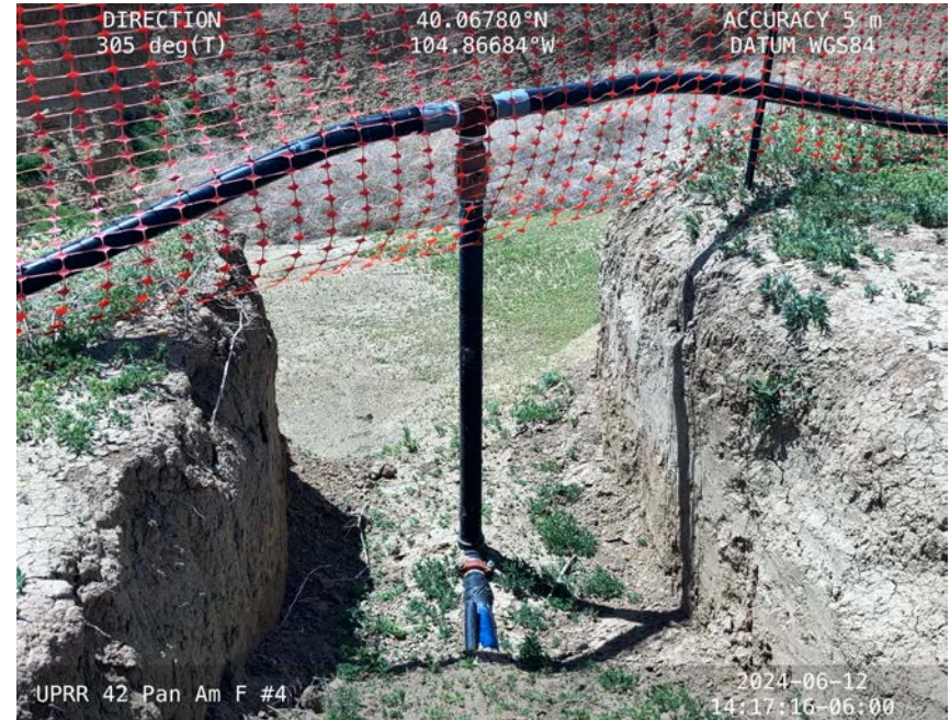
Photo 10 – Fencing does not properly surround excavation
