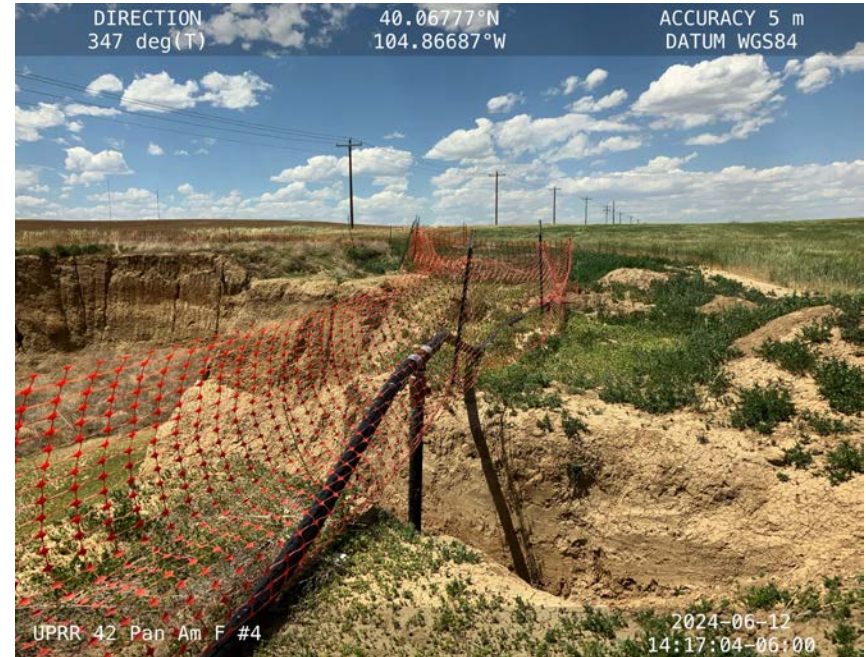
Photo 12 – Fencing does not properly surround excavation
