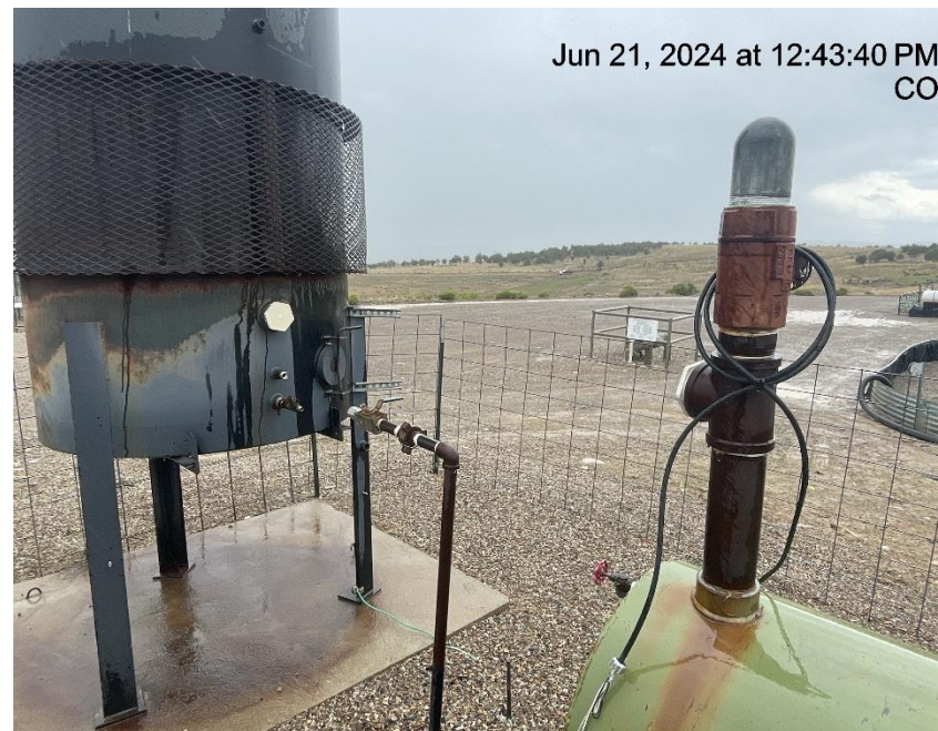
Photo # 955 Unused Equipment/ECD disconnected
