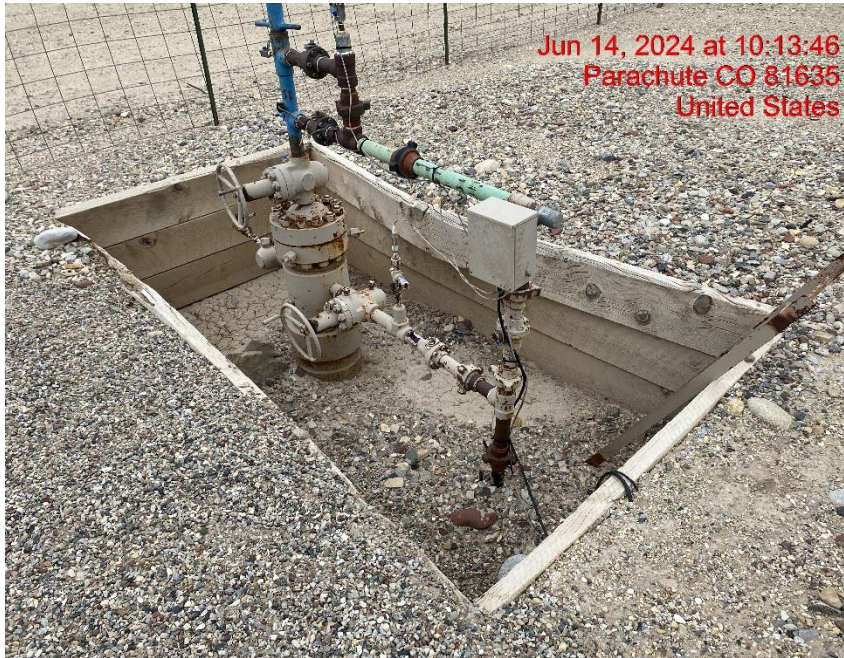
Open Wellhead Cellar – Photo #01731
