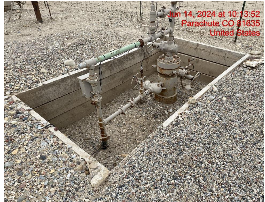
Open Wellhead Cellar – Photo #01732
