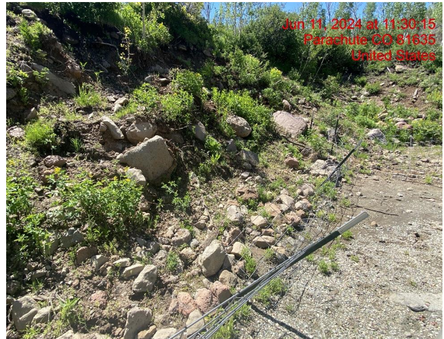
Cut Slope Degradation/Damaged Fencing – Photo #01718
