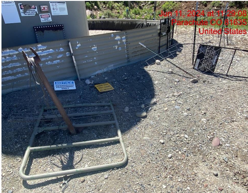
Battery Fencing Damaged – Photo #01715
