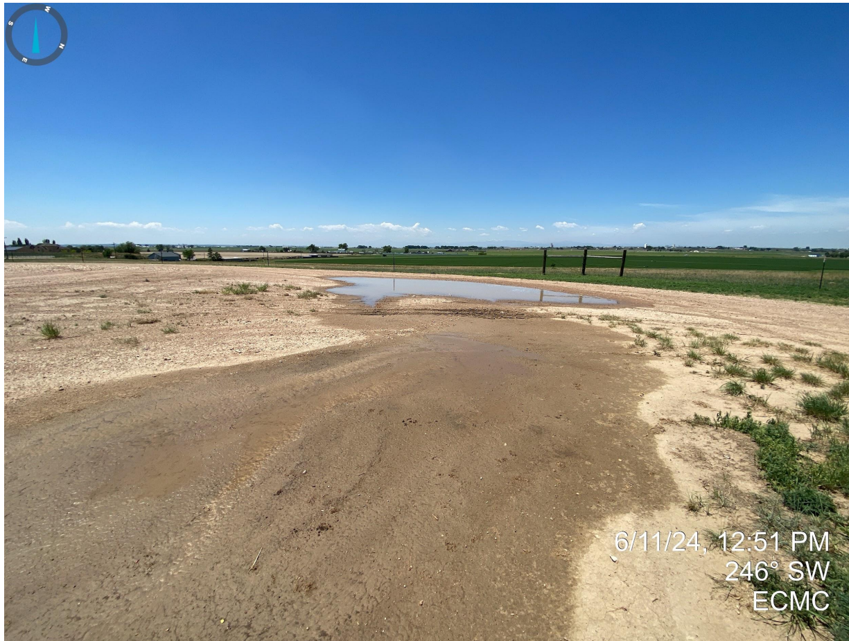
Photo 6. The western portion of the former tank battery location does not appear to have been contoured/graded to prevent the accumulation of stormwater on the access road.
