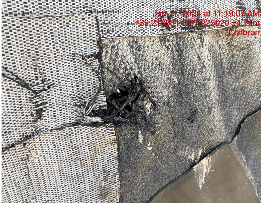
Hole in liner - Photo #02358
