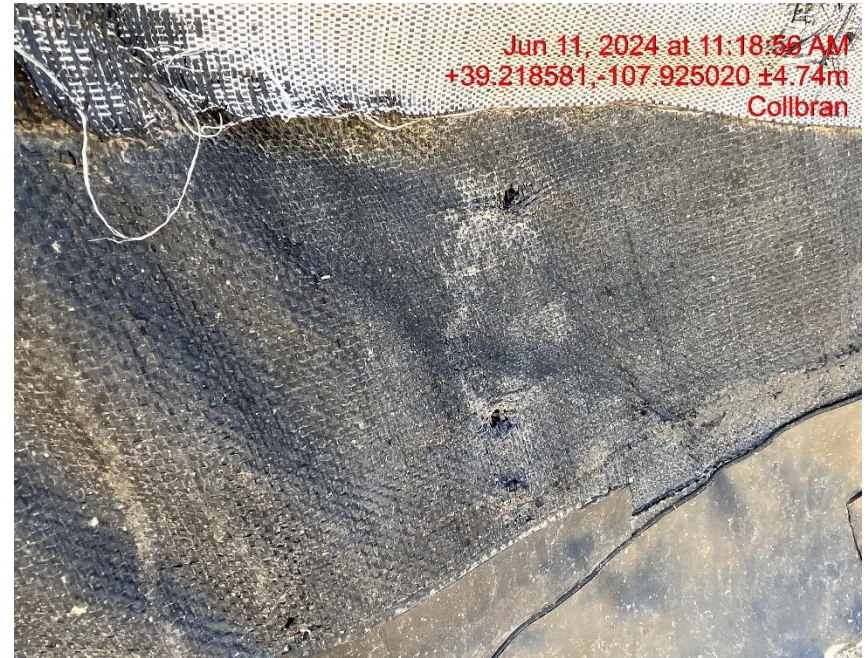
Holes in liner - Photo #02357
