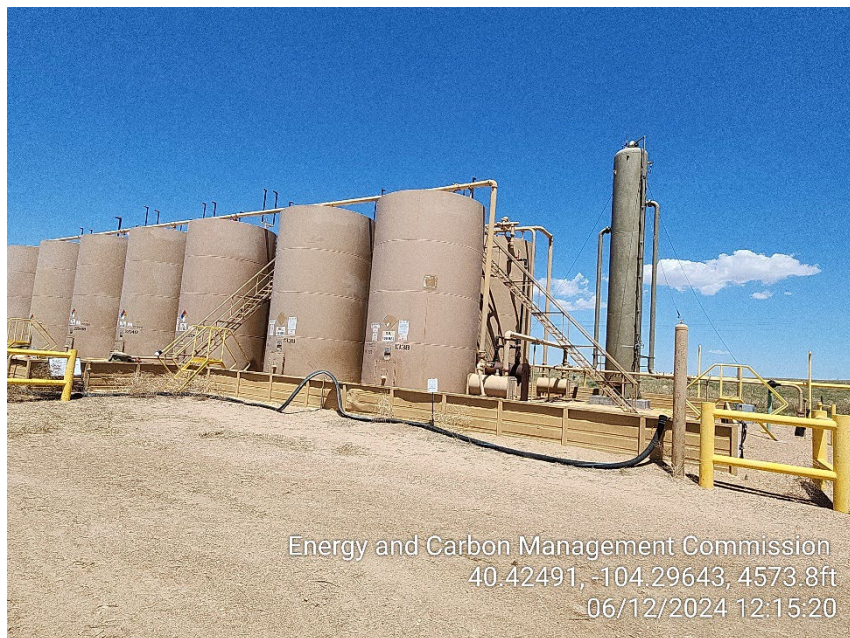
Photo 3 – Tank Battery
