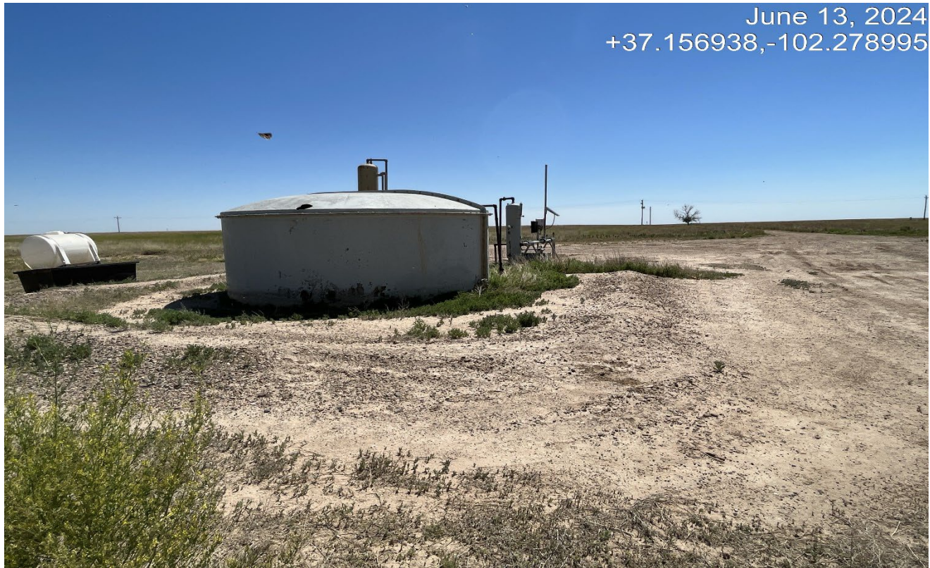
Photo 4. The berm around the tank is worn down and needs to be rebuilt.
