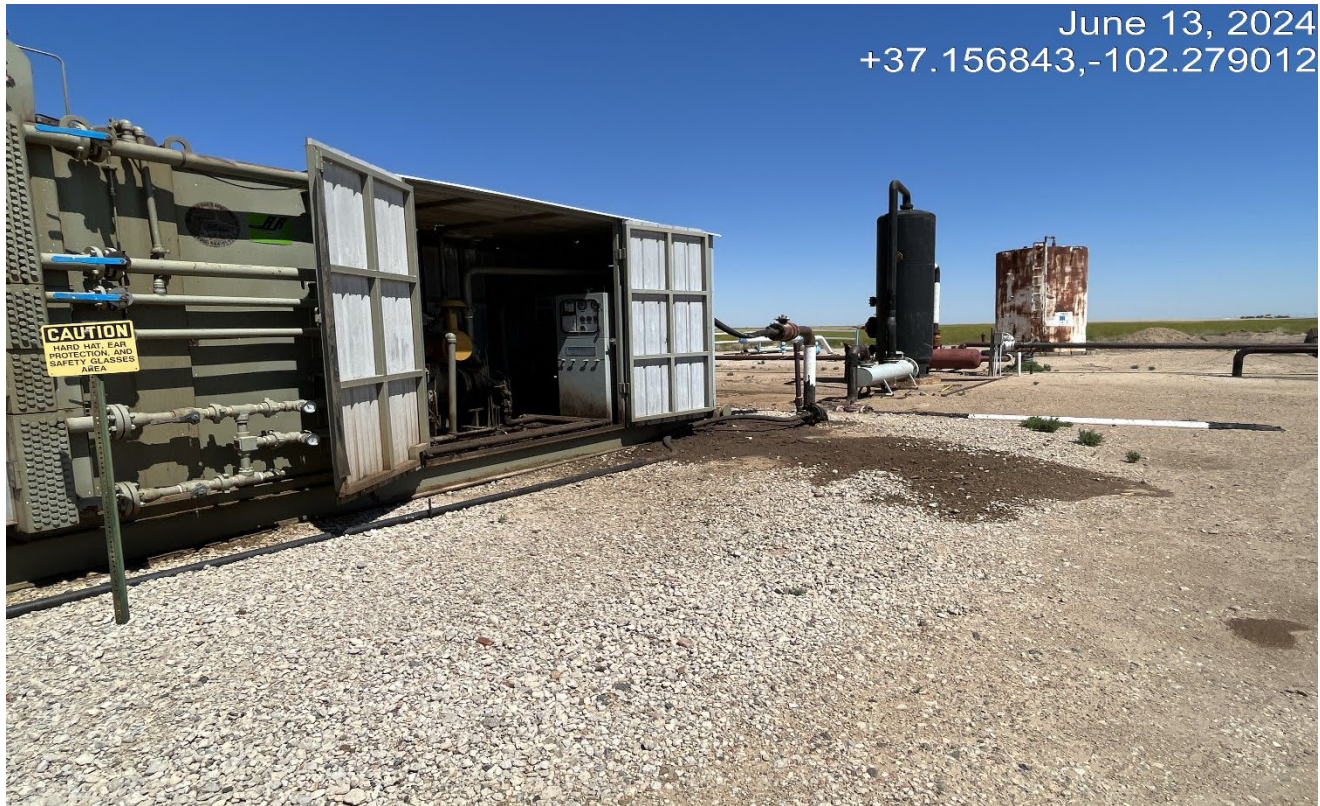
Photo 7. Facing toward the engine compressor. There is oil stained soils from the compresoor leaking lube oil.
