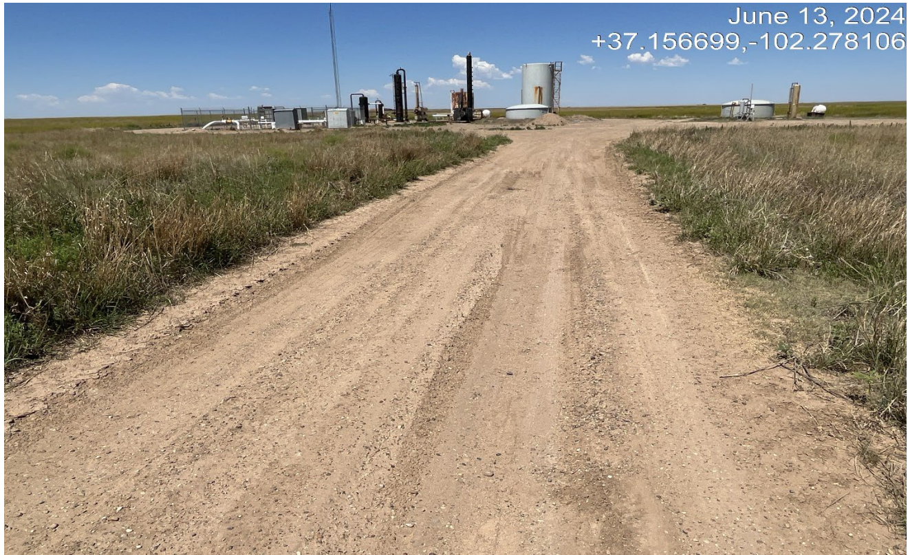
Photo 1. Facing east along the access road. There is rutted areas along the road that need maintenance.
