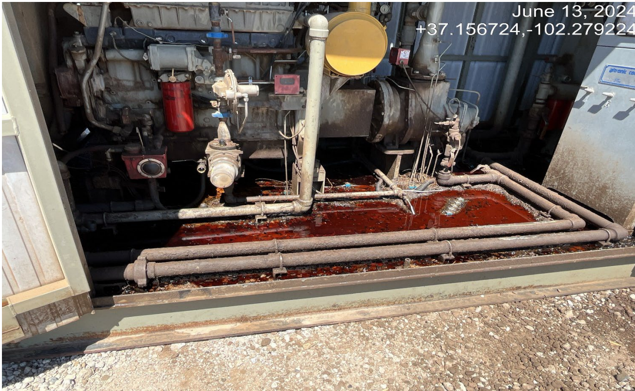
Photo 8. There is oily fluids in the engine skid that must be cleaned up.
