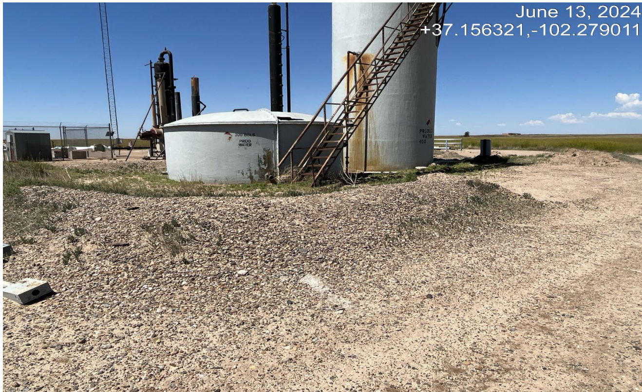
Photo 5. Facing southwest. There is no berm around the north and west side of the tank battery to prevent a spill. The labels on the tanks are faded and worn off.
