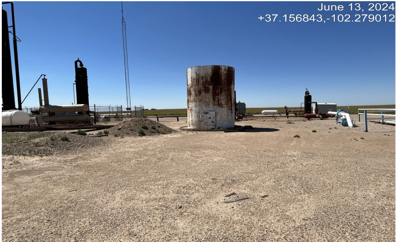
Photo 6. Facing south at the location. There is no secondary containment at the tank shown in the photo.
