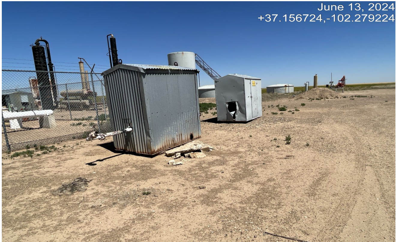
Photo 9. There are two unused meter sheds that need to be removed per Rule 606.
