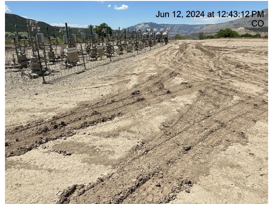
Photo # 649 Lack of stabilization/compaction
