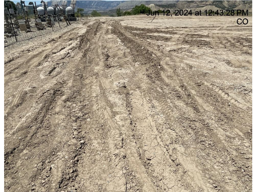
Photo # 651 Lack of stabilization/compaction
