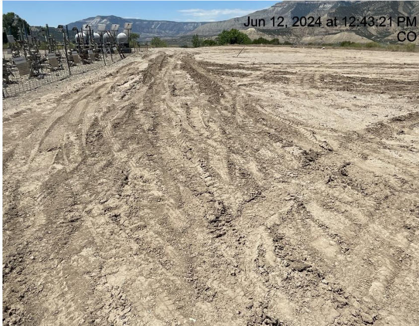
Photo # 650 Lack of stabilization/compaction
