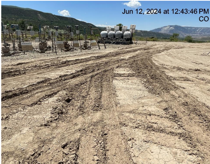
Photo # 654 Lack of stabilization/compaction
