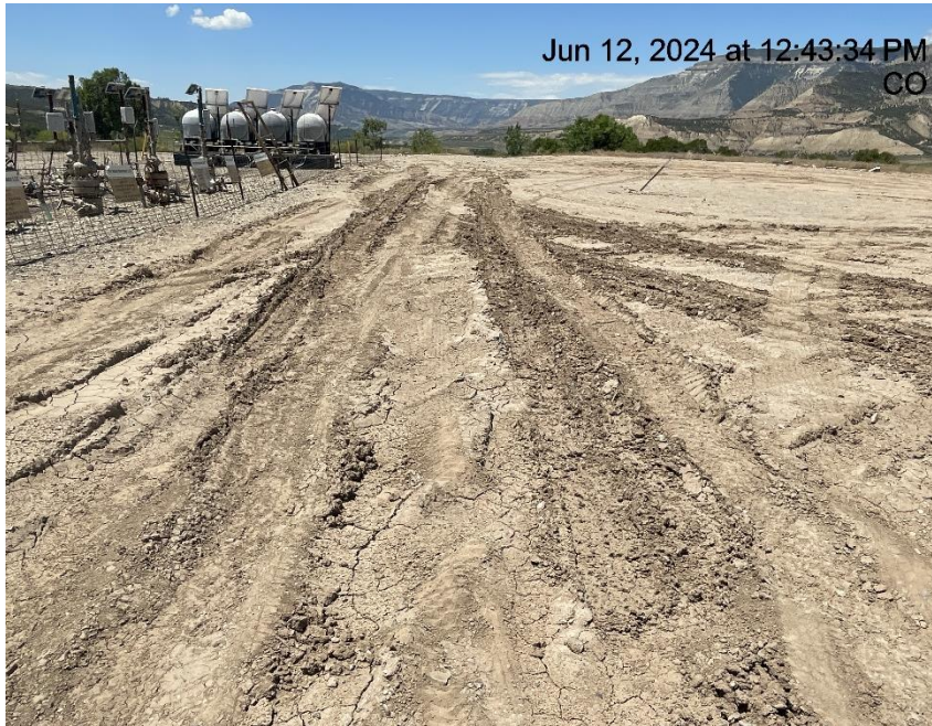
Photo # 652 Lack of stabilization/compaction
