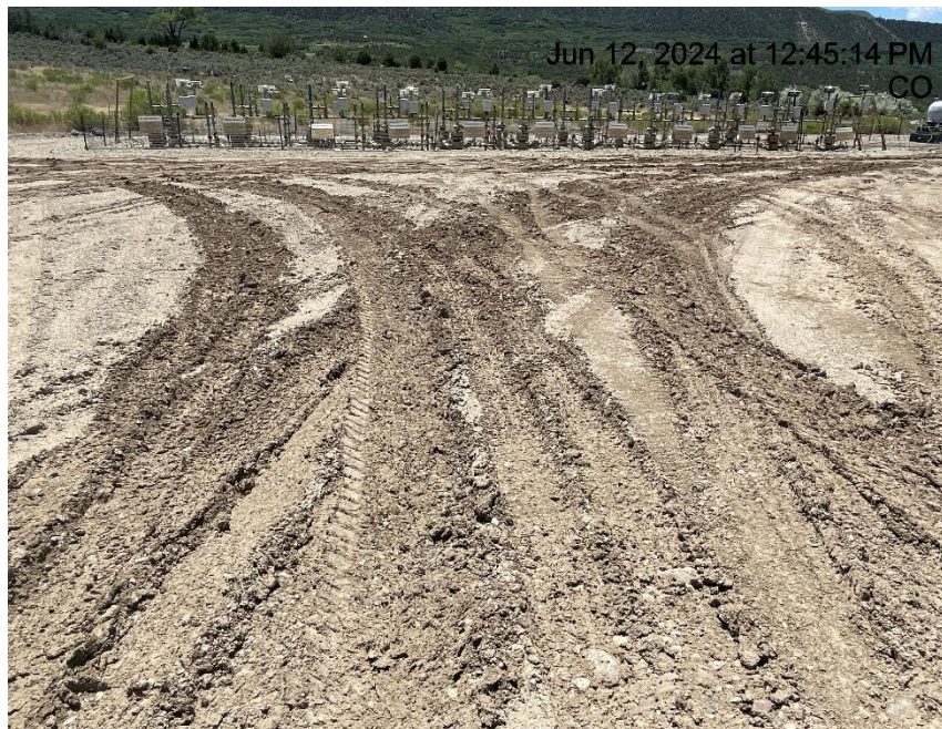
Photo # 658 Lack of stabilization/compaction
