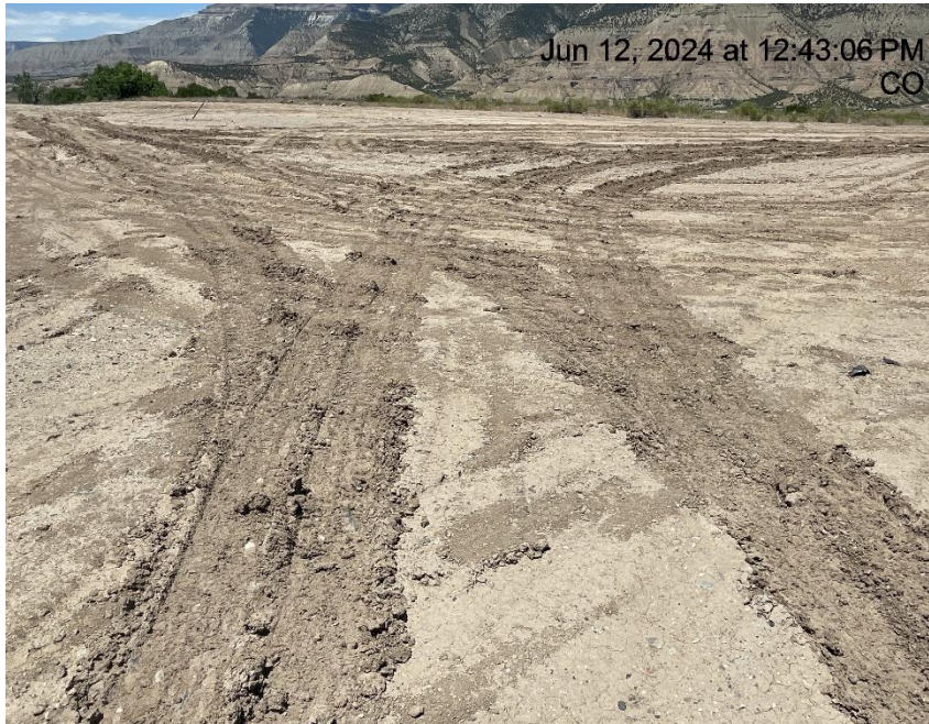
Photo # 648 Lack of stabilization/compaction
