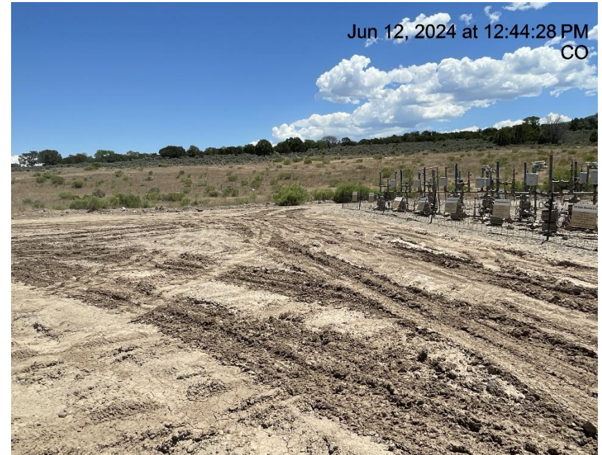
Photo # 657 Lack of stabilization/compaction
