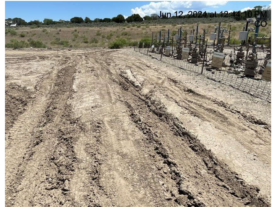
Photo # 655 Lack of stabilization/compaction
