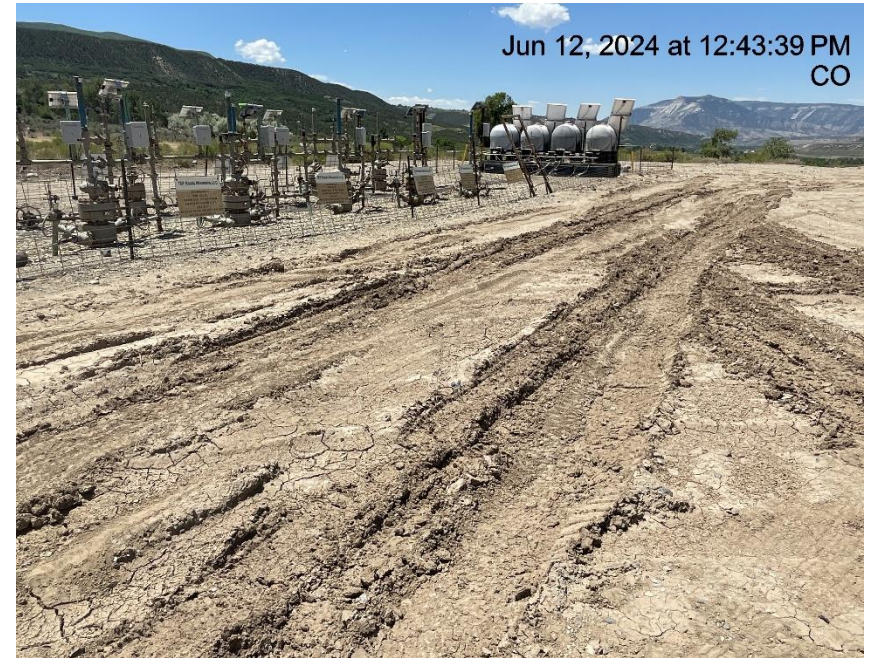
Photo # 653 Lack of stabilization/compaction
