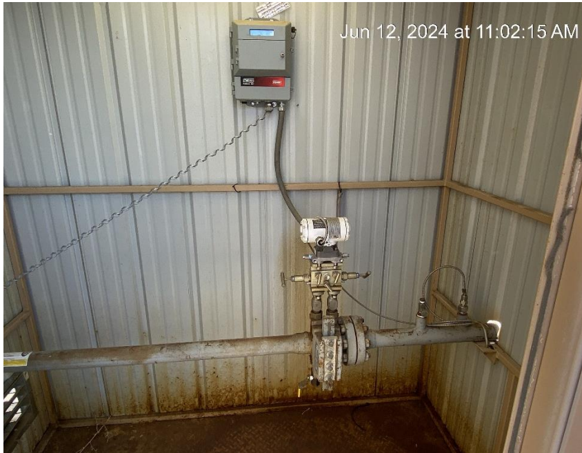
No gas meter calibration visible
