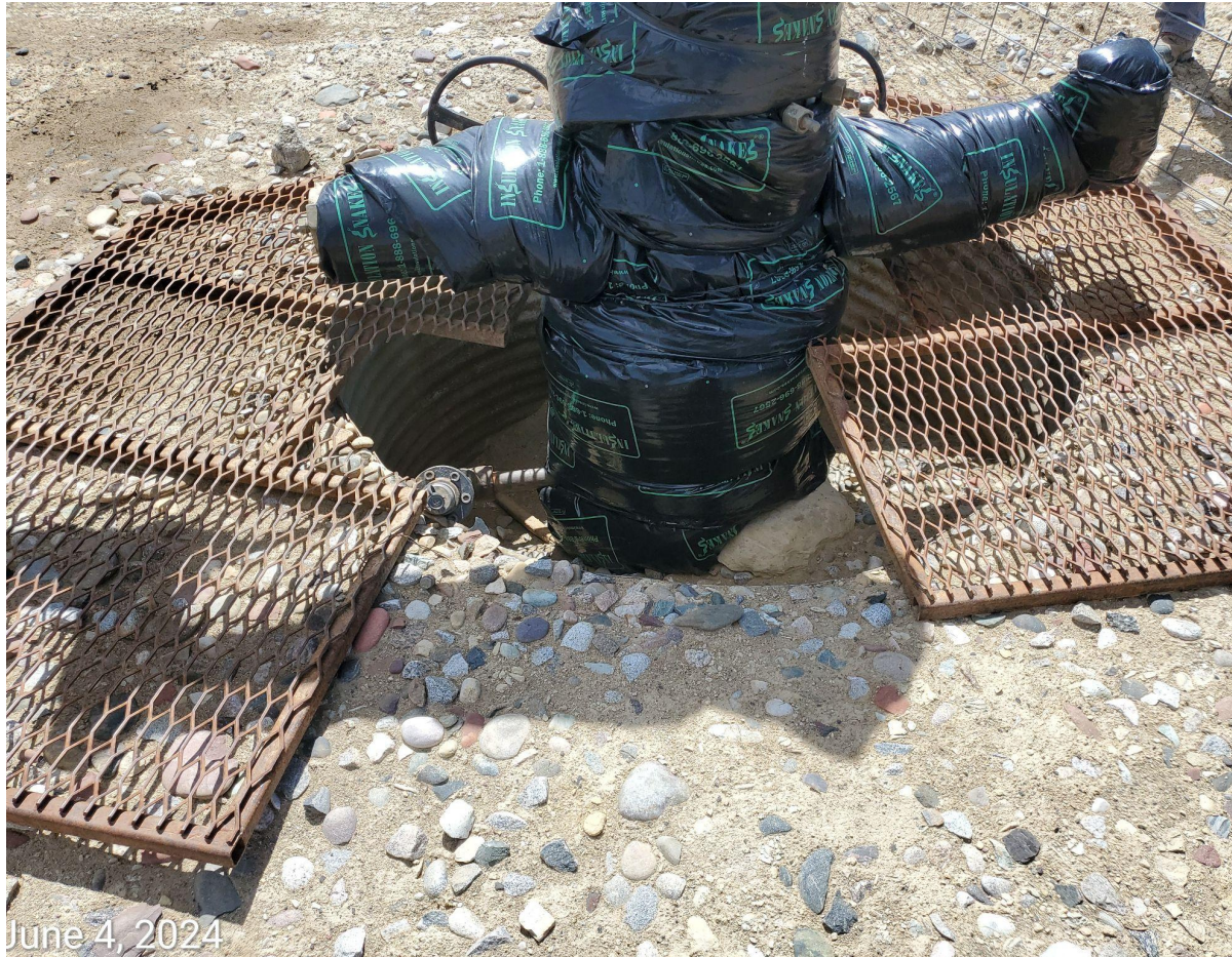
Photo 2: Cover at cellar no longer appears to adequately fit around well.
