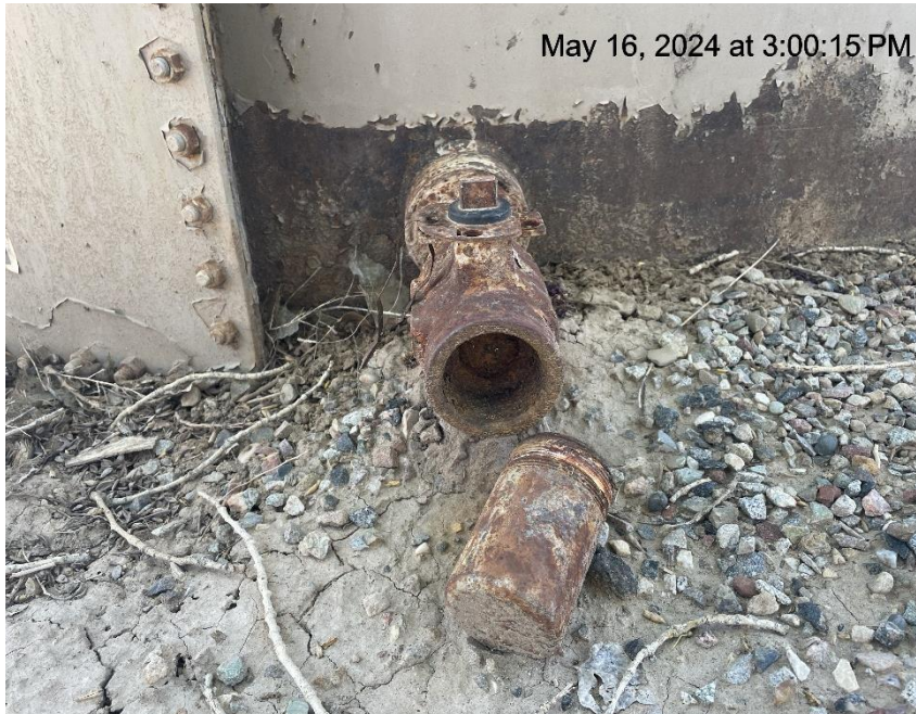
Photo # 7496 From inspection 708903824 conducted on 05/16/2024 Open ended load line
