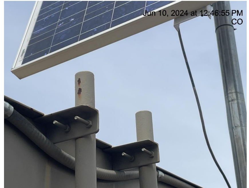
Photo # 161 PRV & rupture disc vent lines do not comply with CECMC pressure safety device rules
