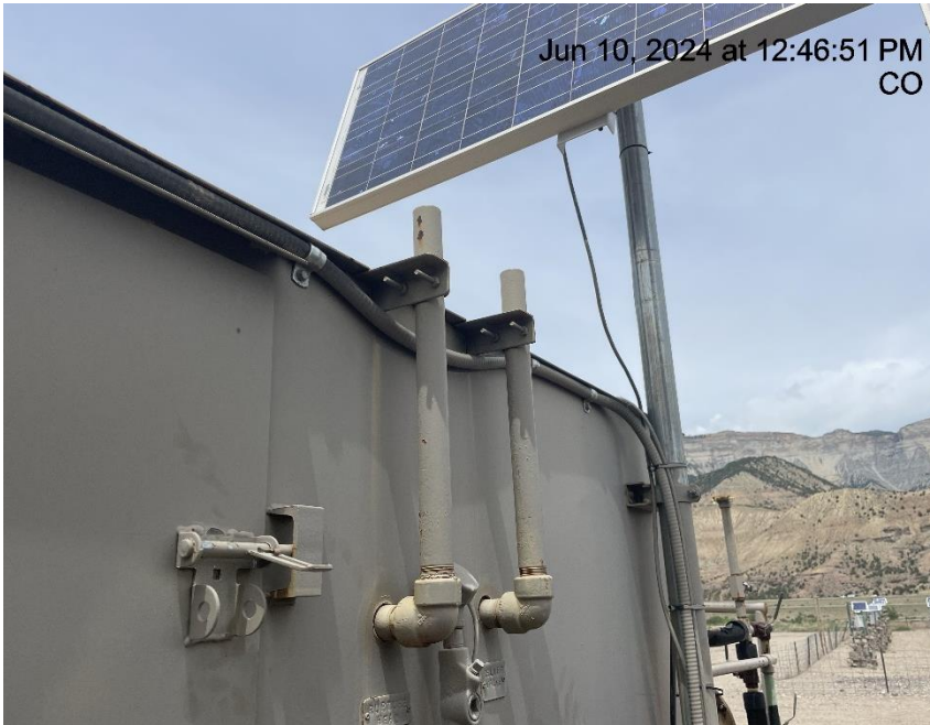
Photo # 160 PRV & rupture disc vent lines do not comply with CECMC pressure safety device rules
