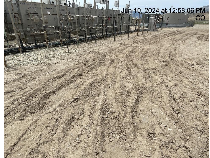
Photo # 165 Lack of stabilization/compaction
