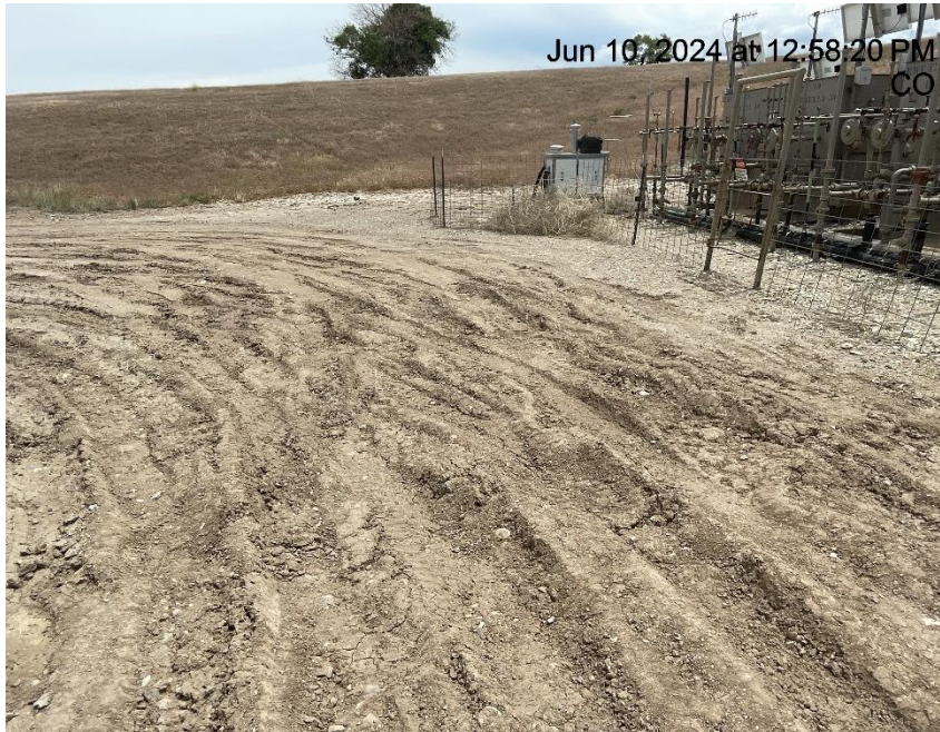
Photo # 166 Lack of stabilization/compaction
