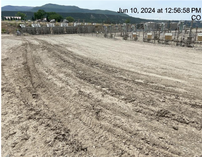
Photo # 162 Lack of stabilization/compaction
