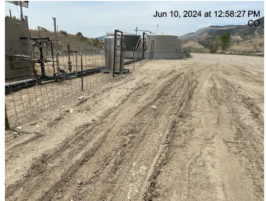
Photo # 167 Lack of stabilization/compaction
