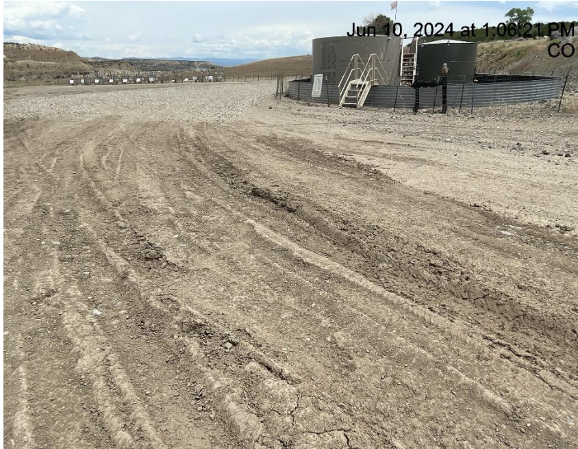
Photo # 168 Lack of stabilization/compaction
