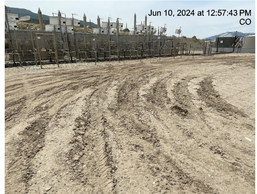
Photo # 163 Lack of stabilization/compaction
