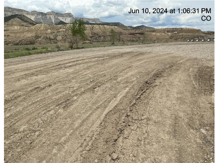
Photo # 169 Lack of stabilization/compaction
