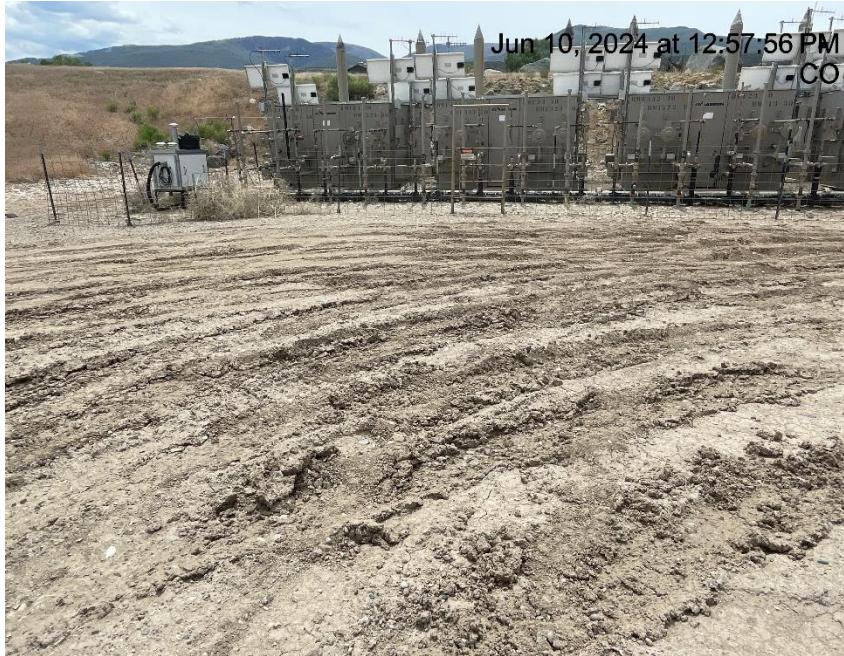
Photo # 164 Lack of stabilization/compaction
