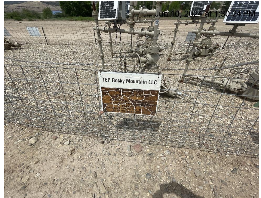
Photo # 220 Wellhead sign weathered & cracking/sign is becoming illegible & does not comply with CECMC rules
