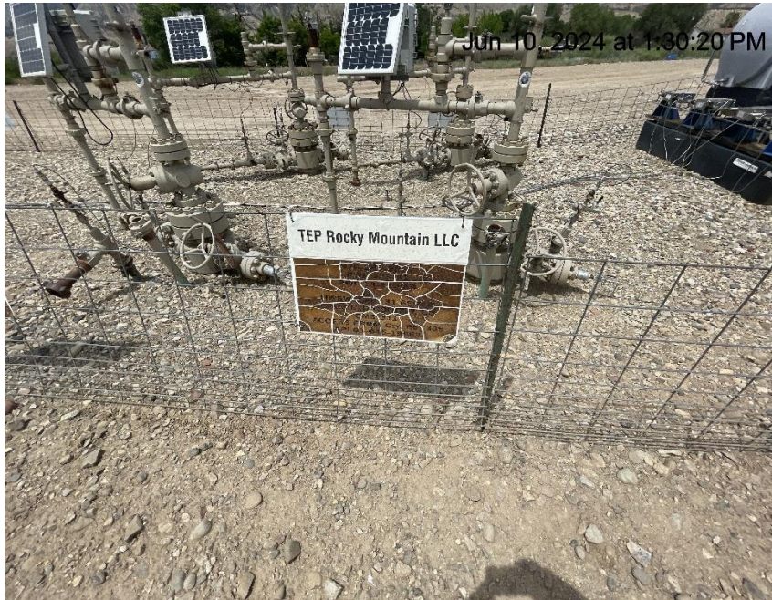
Photo # 219 Wellhead sign weathered & cracking/sign is becoming illegible & does not comply with CECMC rules
