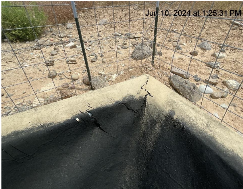
Photo # 225 Small amount of damage near top of secondary containment liner
