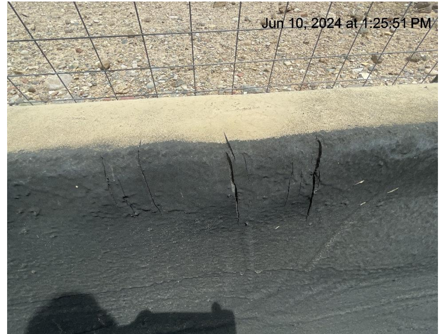
Photo # 226 Small amount of damage near top of secondary containment liner
