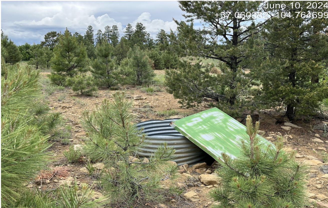
Photo 2. This culvert is not covered along the flowline. The lid needs to be kept on to prevent wildlife entry..
