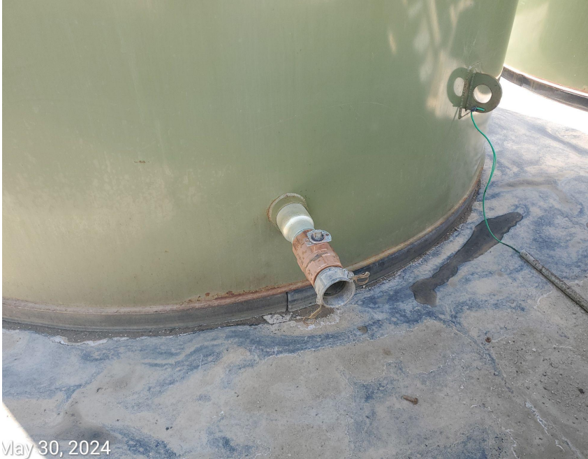
Photo 5: Photos examples showing lines at tanks missing required cap/plug.
