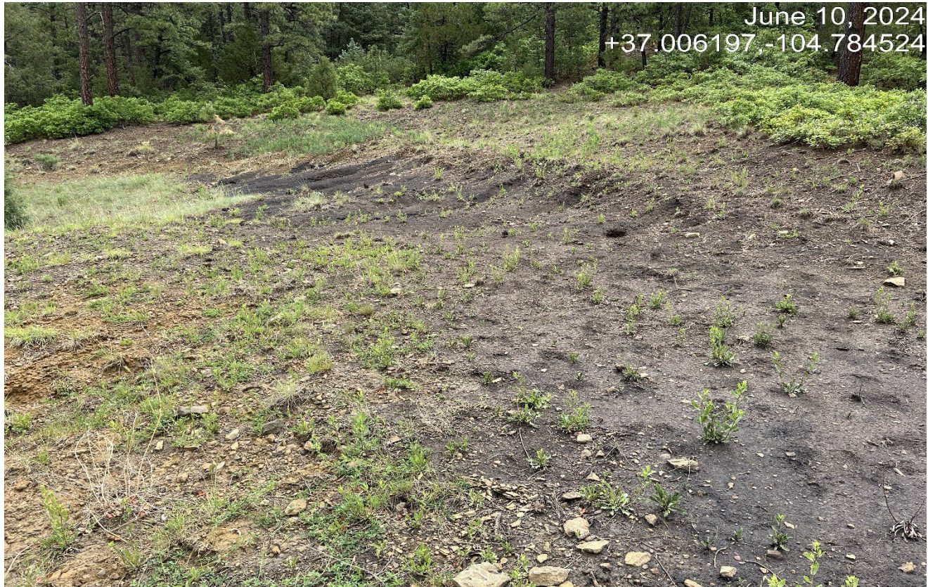
Photo 5. The top of the cut slope need to be stabilized and may require a run-on ditch or other BMP's.
