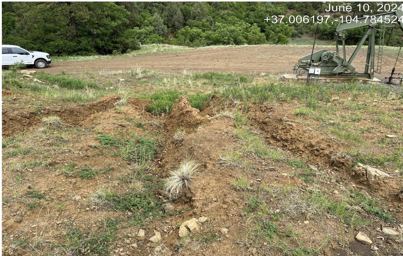
Photo 6. Facing northwest along the cut slope. There are erosion channels that must be repaired and stabilized.
