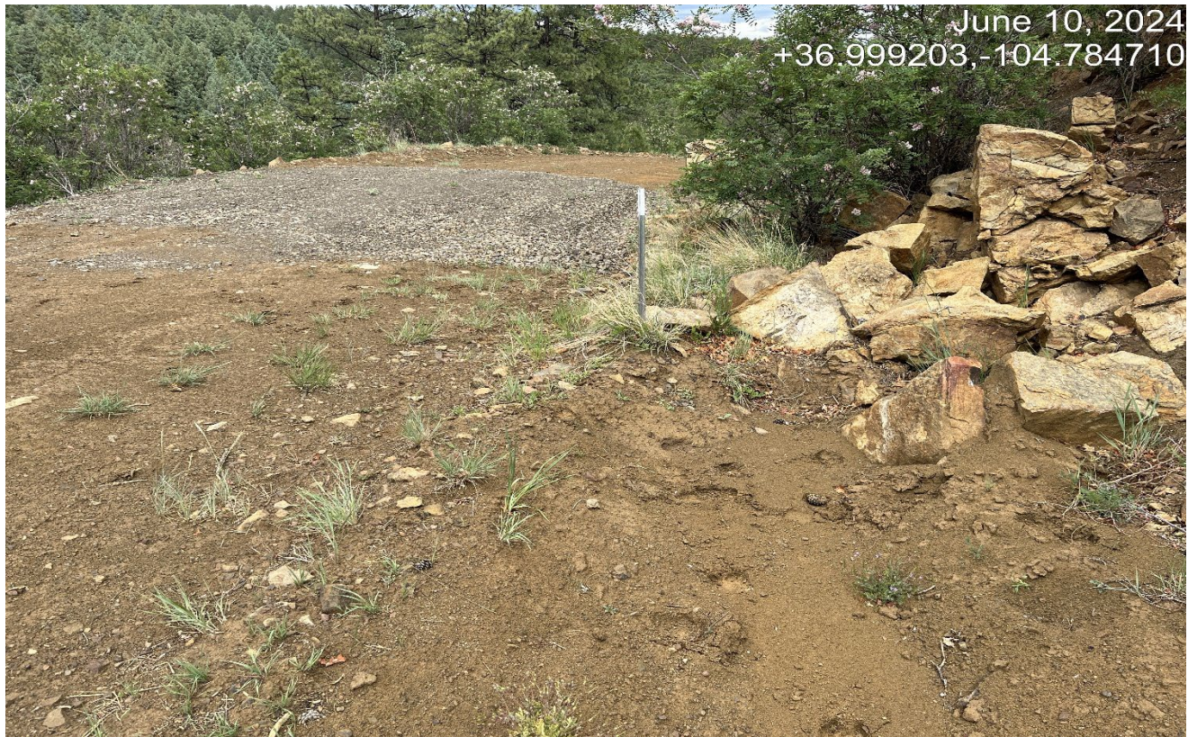
Photo 1. Facing northeast along the access road. The culvert has filled in with sediment and needs to be cleaned out.
