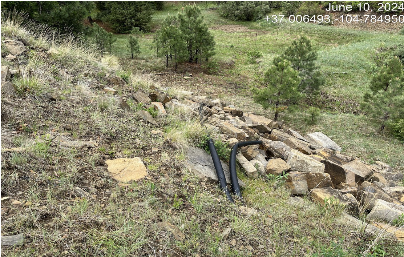
Photo 7. There are black polylines at the fill slope that must removed.
