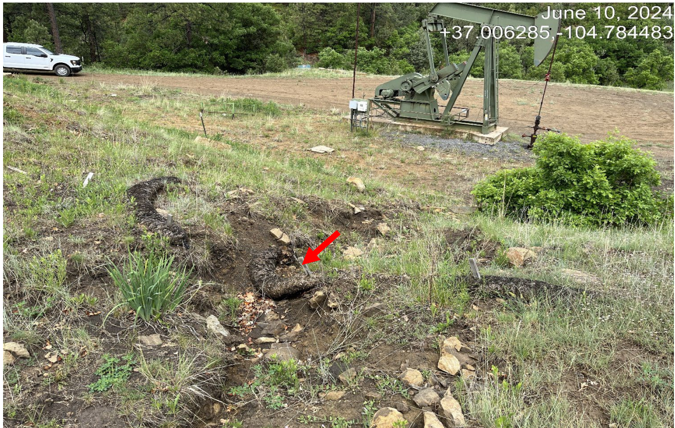
Photo 4. Facing northwest the cut slope. There are erosion channels that need to be repaired. The wattles at red arrow has failed.
