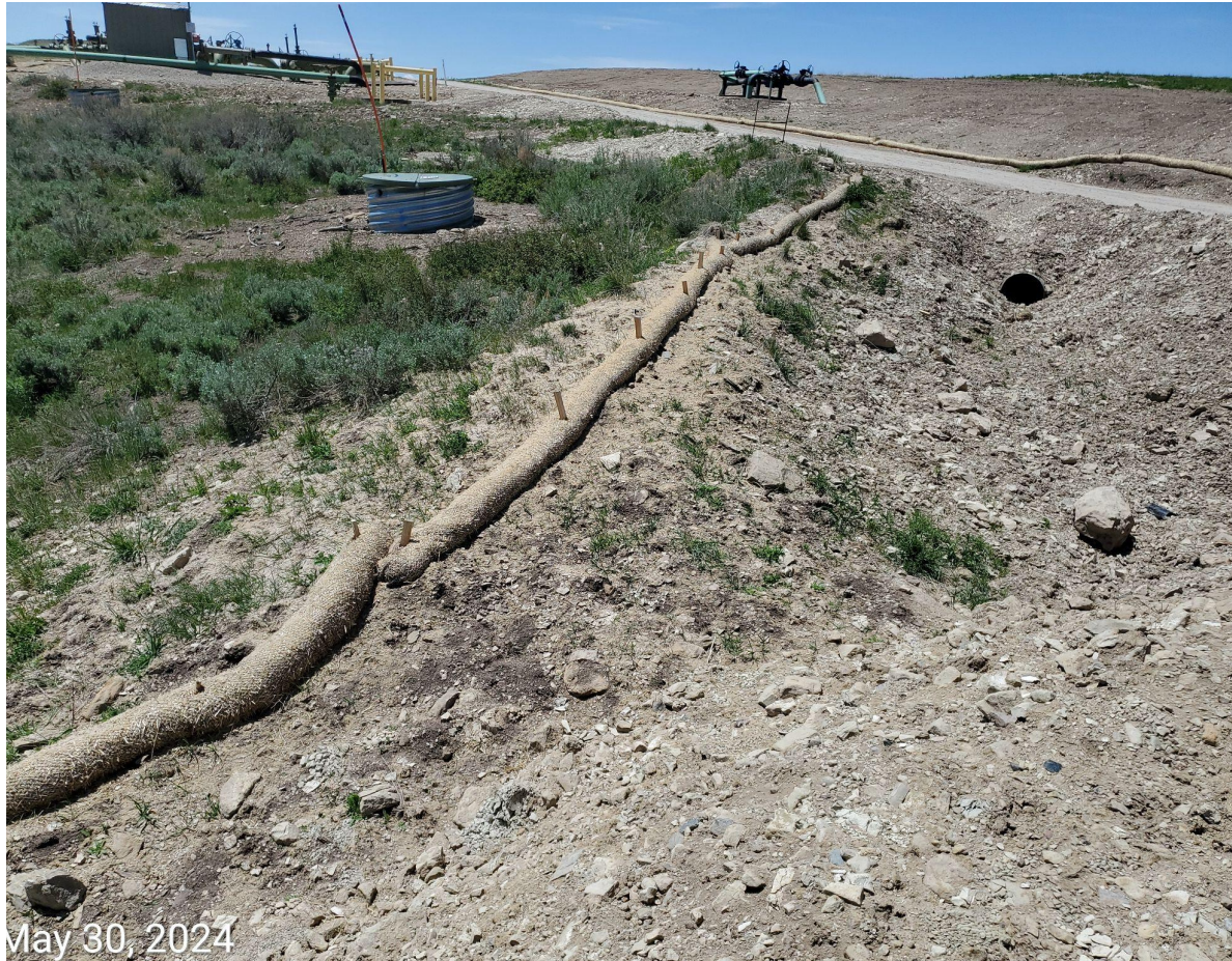
Photo 7: Photos examples showing erosion logs on the Location that have not been properly back-filled per good engineering practice.
