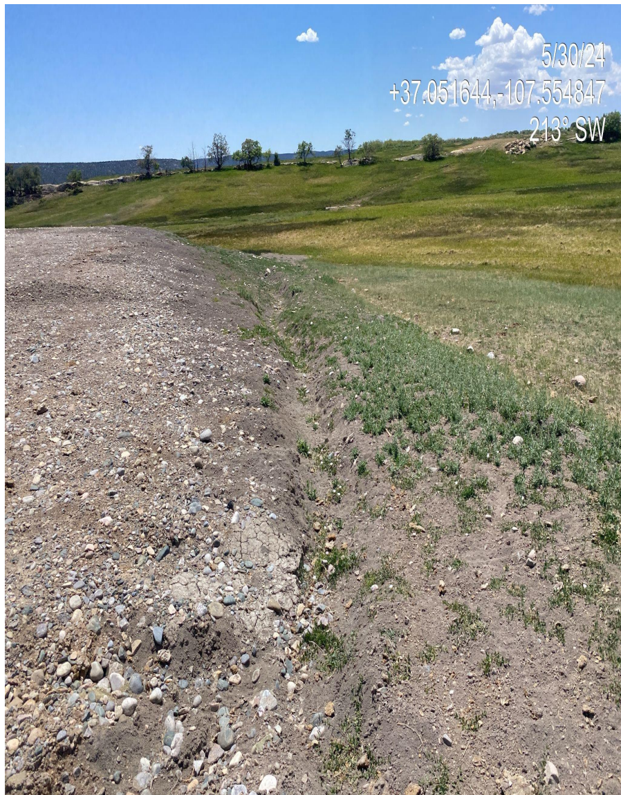
Photo 2. View of the diversion and evidence of sediment transport/deposition. Reseeding appears unsuccessful as interim reclamation areas to the south are dominated by weedy vegetation.
