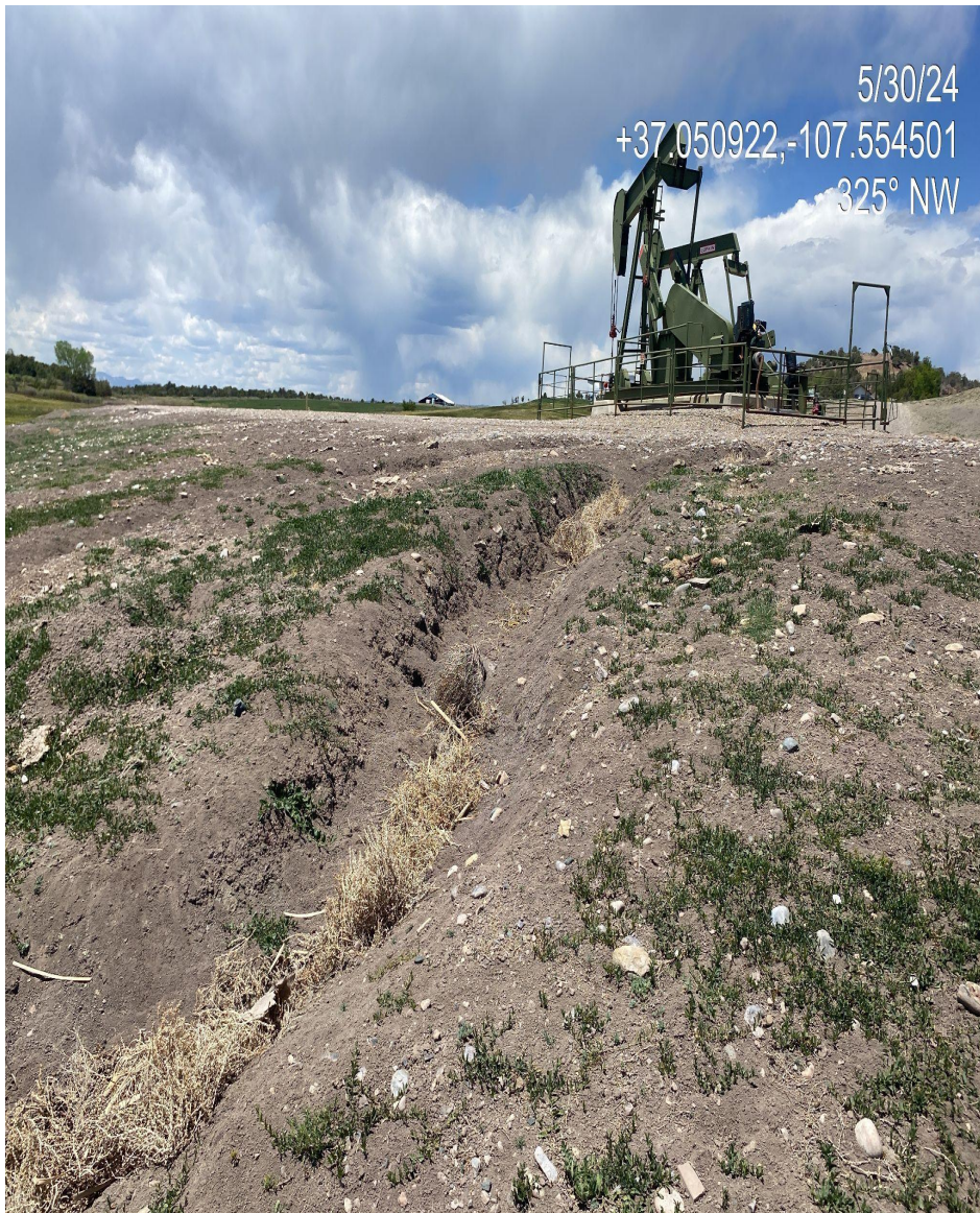
Photo 4. Additional photos of gully erosion and evidence of sediment transport off of location in the southern interim reclamation area.
