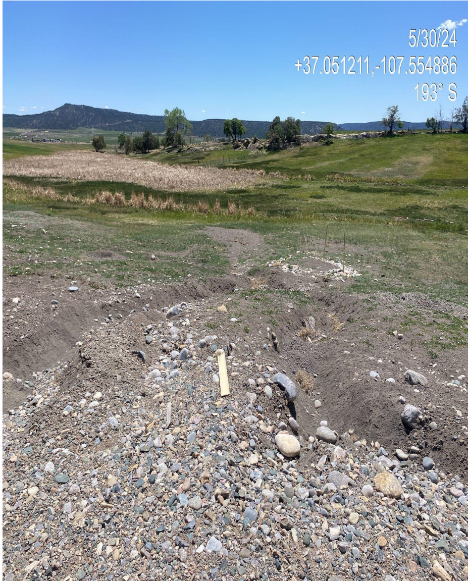
Photo 3. Sever gully erosion observed forming throughout the southern portions of the interim reclamation area, additional stabilization is needed.
