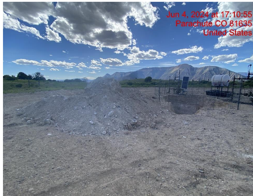
Unprotected Soil Stockpile – Photo #01551
