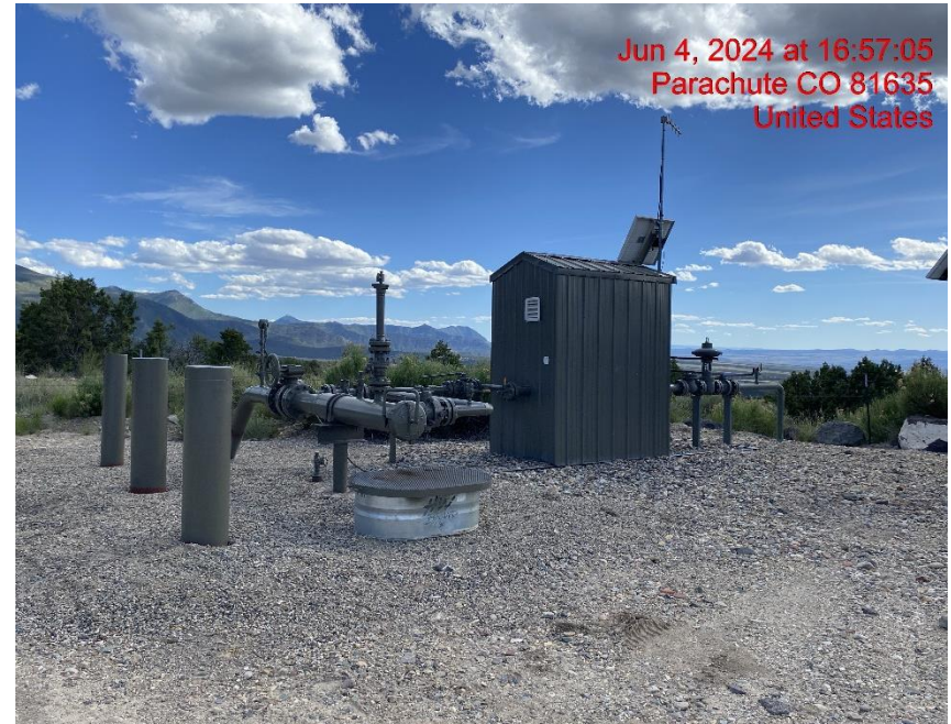
Gas Meter/Pig Station – Photo #01537
