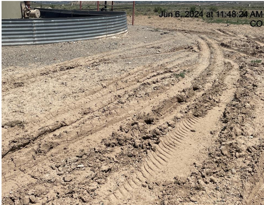
Photo # 9978 Lack of stabilization/compaction
