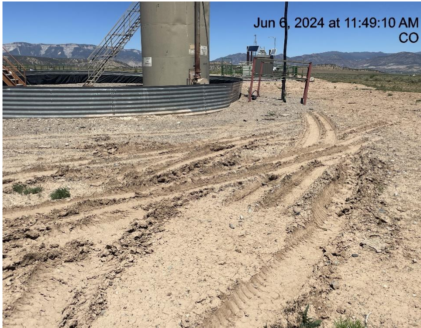
Photo # 9980 Lack of stabilization/compaction
