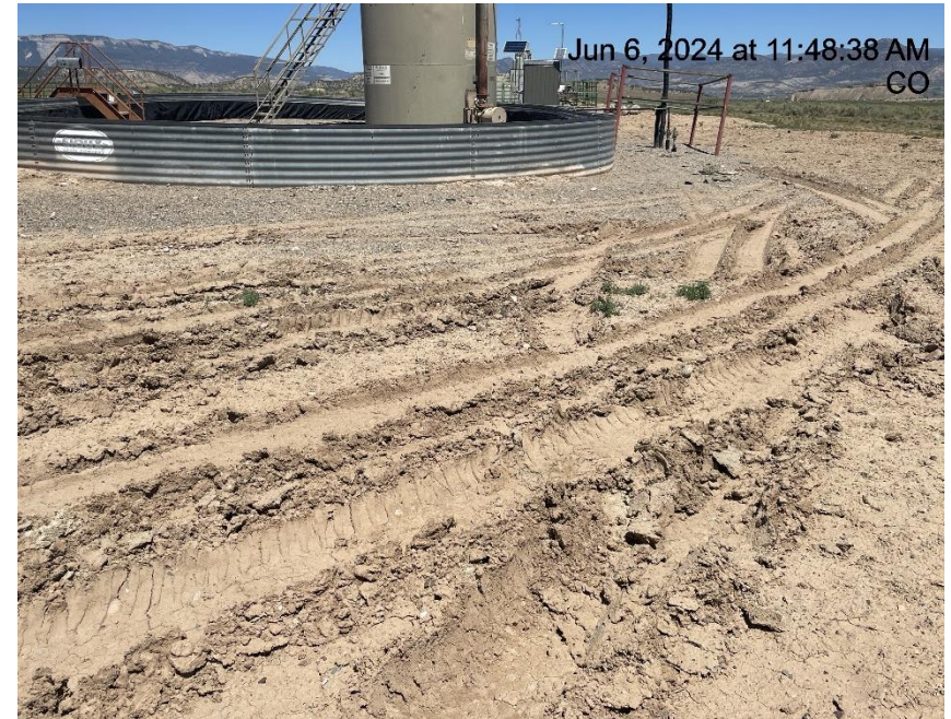
Photo # 9979 Lack of stabilization/compaction
