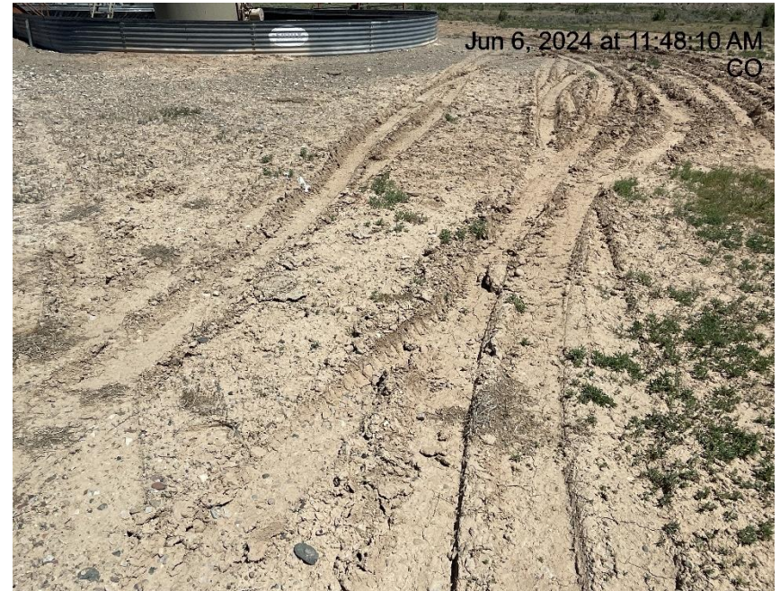
Photo # 9975 Lack of stabilization/compaction
