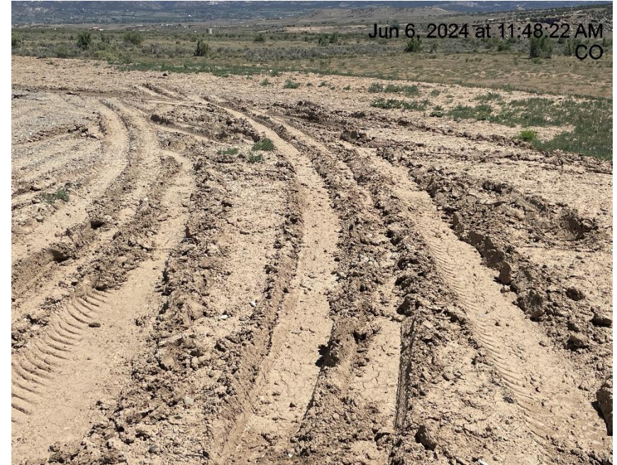
Photo # 9977 Lack of stabilization/compaction
