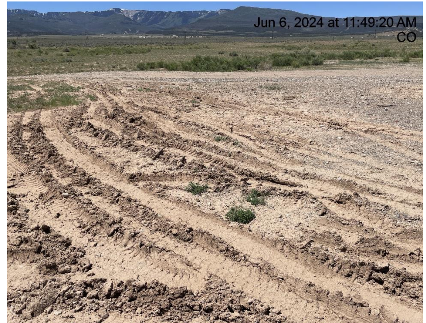
Photo # 9981 Lack of stabilization/compaction
