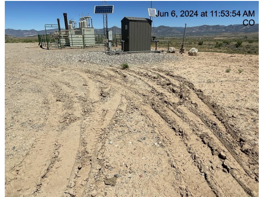
Photo # 9983 Lack of stabilization/compaction
