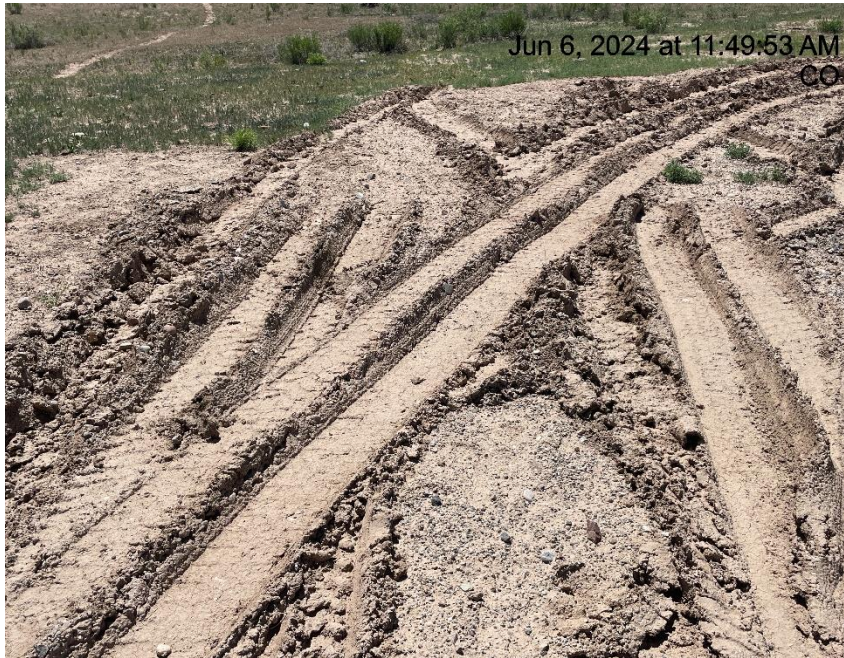
Photo # 9974 Lack of stabilization/compaction
