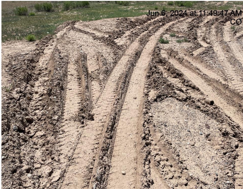
Photo # 9982 Lack of stabilization/compaction
