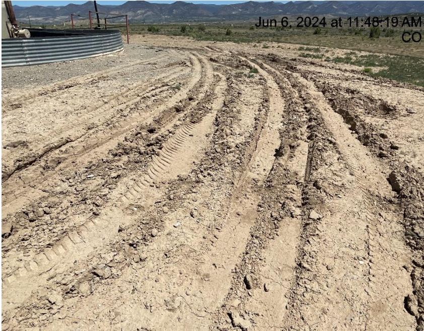
Photo # 9976 Lack of stabilization/compaction
