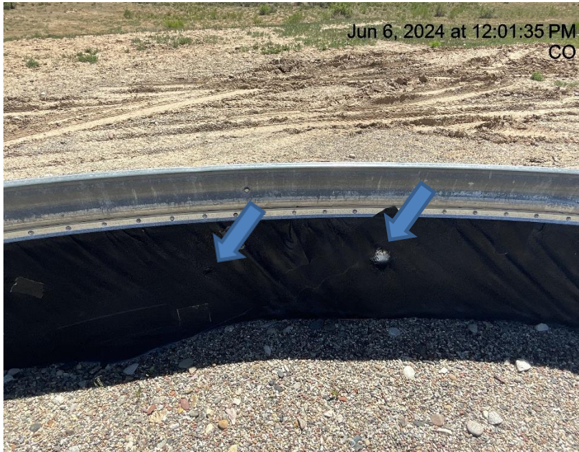
Photo # 9957 Holes in liner/liner needs maintenance
