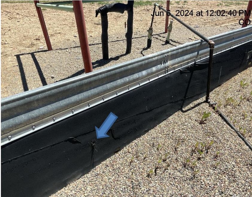
Photo # 9967 Hole in liner/liner needs maintenance
