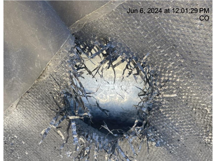
Photo # 9956 Hole in liner/liner needs maintenance
