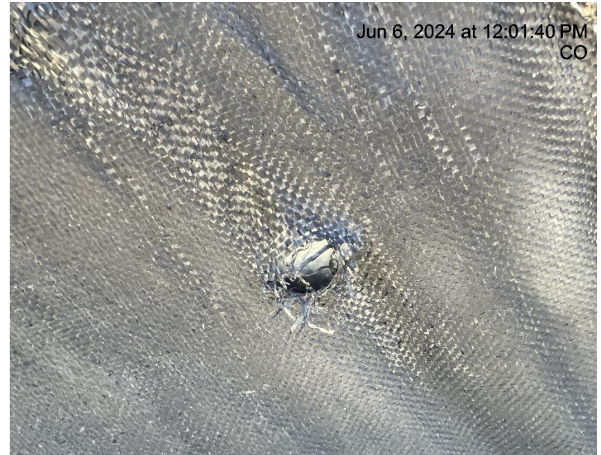
Photo # 9958 Hole in liner/liner needs maintenance
