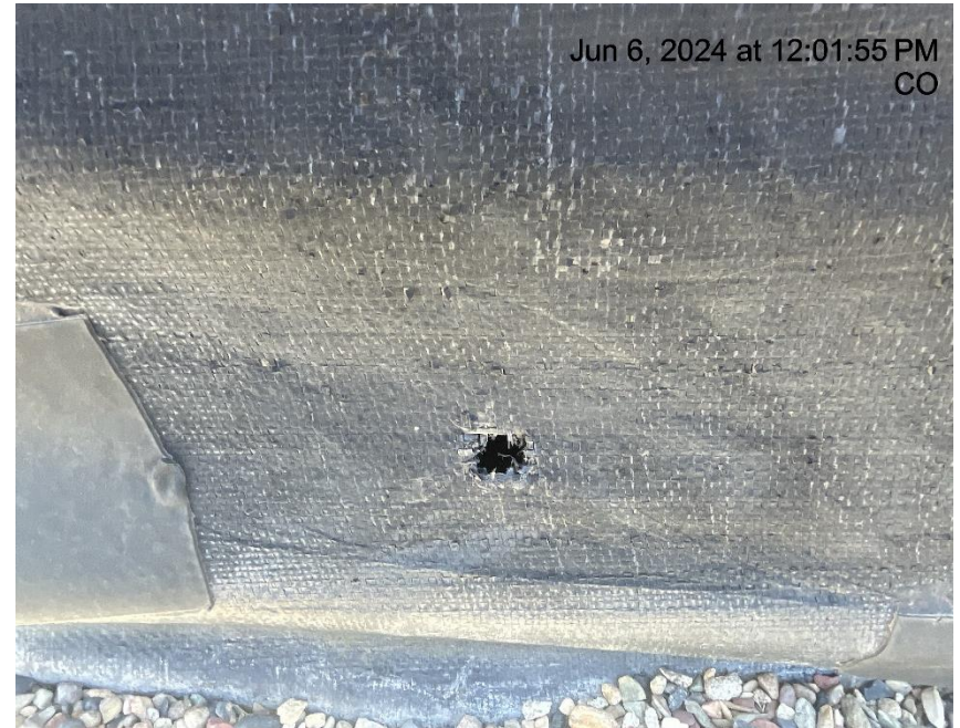
Photo # 9960 Hole in liner/liner needs maintenance
