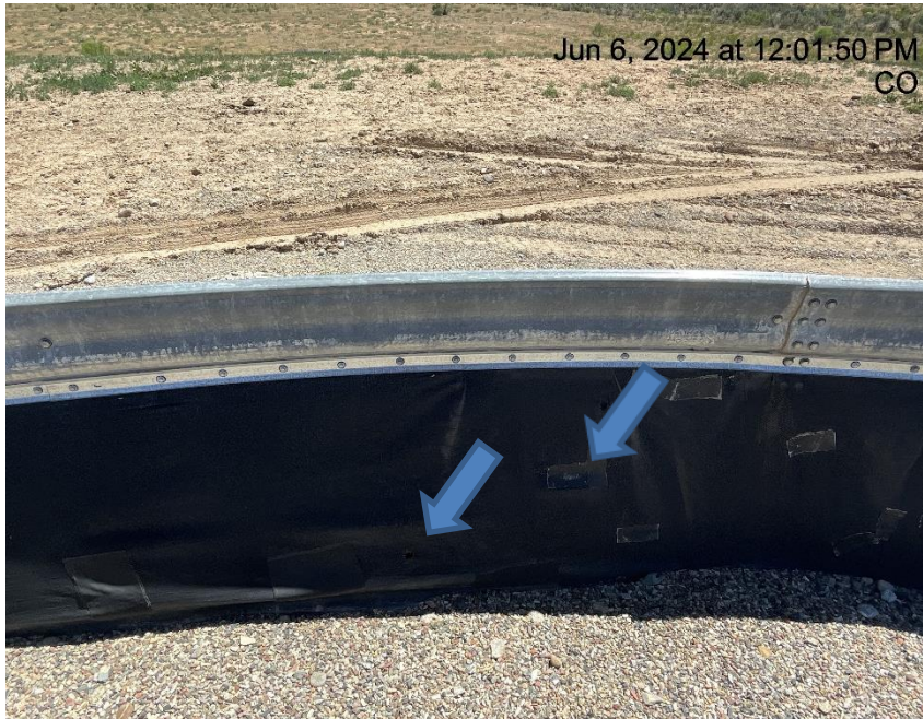
Photo # 9959 Holes in liner/liner needs maintenance
