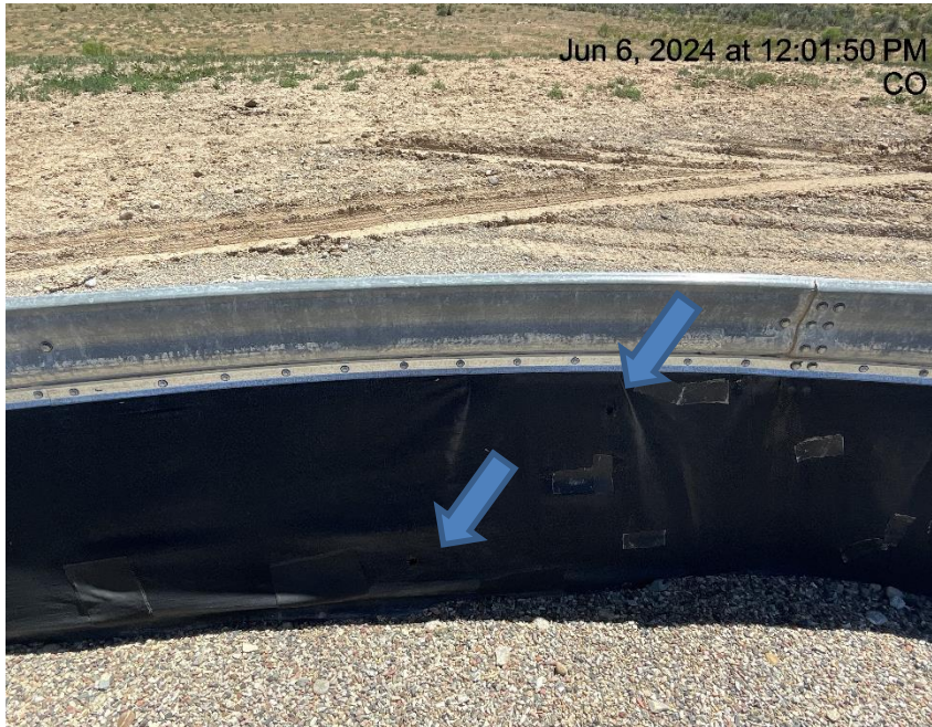
Photo # 9961 Holes in liner/liner needs maintenance
