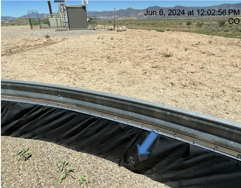
Photo # 9969 Hole in liner/liner needs maintenance
