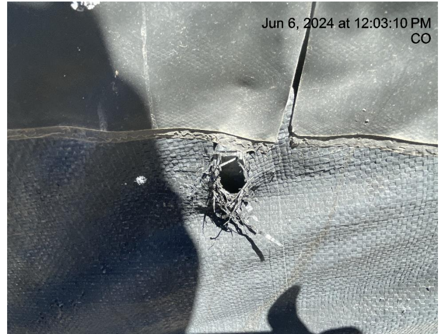
Photo # 9972 Hole in liner/liner needs maintenance
