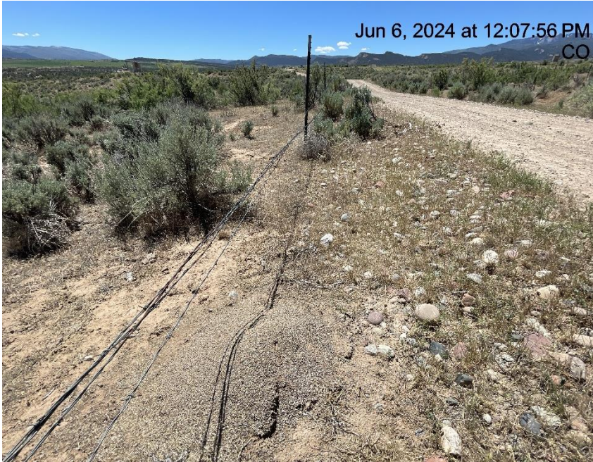
Photo # 9951 Barbed wire fence needs maintenance/wildlife hazard
