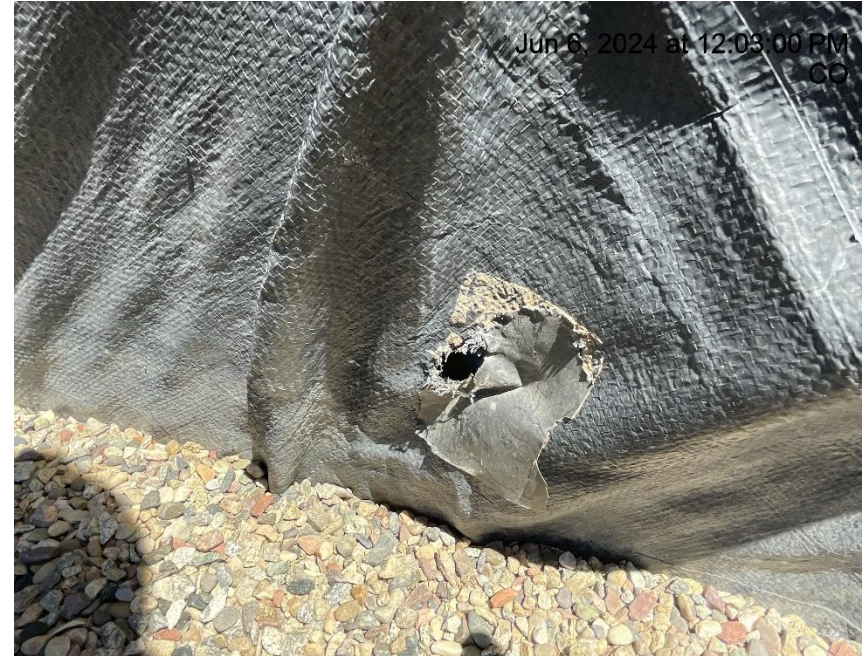
Photo # 9970 Hole in liner/liner needs maintenance
