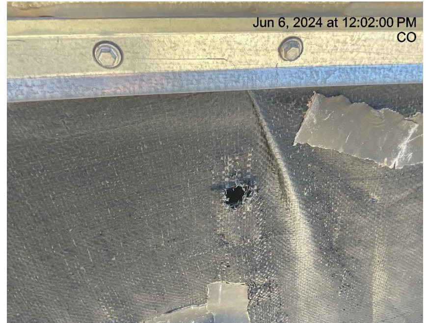
Photo # 9962 Hole in liner/liner needs maintenance
