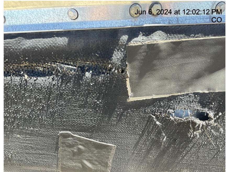
Photo # 9964 Holes in liner/liner needs maintenance
