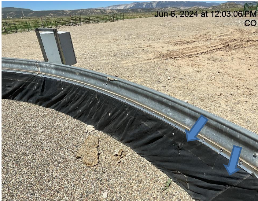
Photo # 9971 Holes in liner/liner needs maintenance
