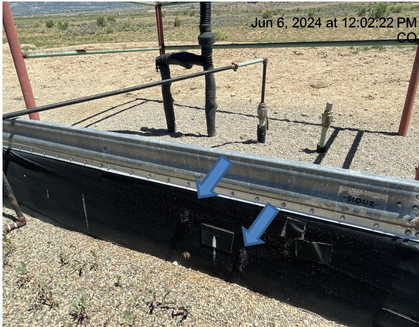
Photo # 9965 Holes in liner/liner needs maintenance
