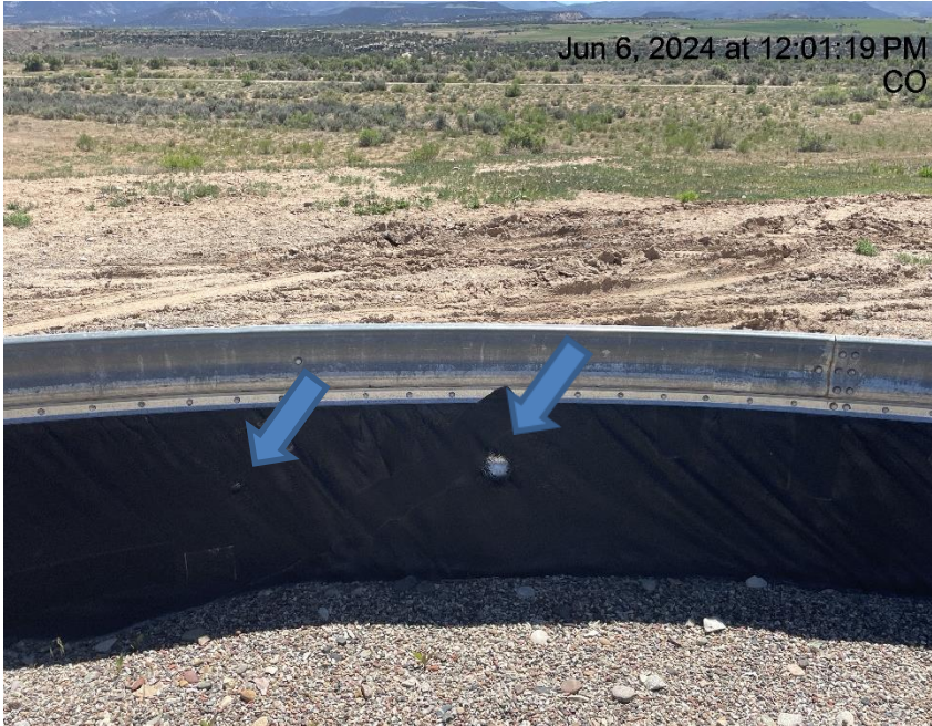
Photo # 9955 Holes in liner/liner needs maintenance
