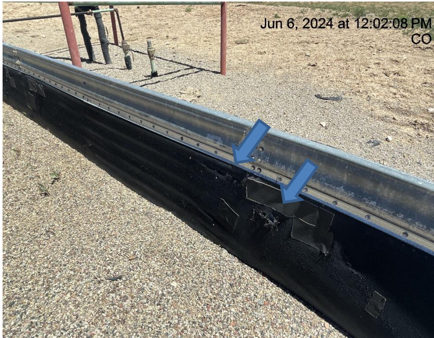
Photo # 9963 Holes in liner/liner needs maintenance
