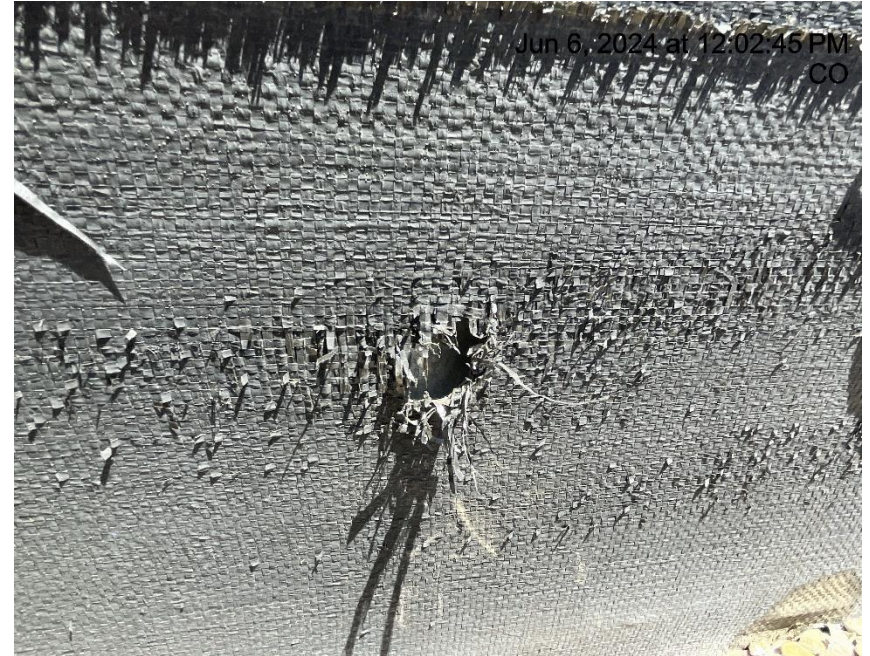
Photo # 9968 Hole in liner/liner needs maintenance
