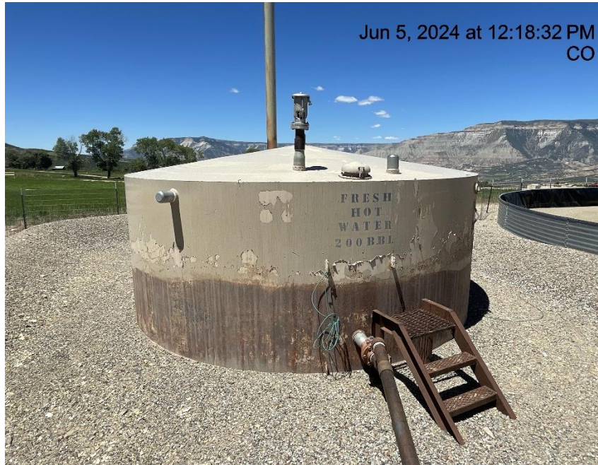
Photo # 9564 Tank lacks required labeling
