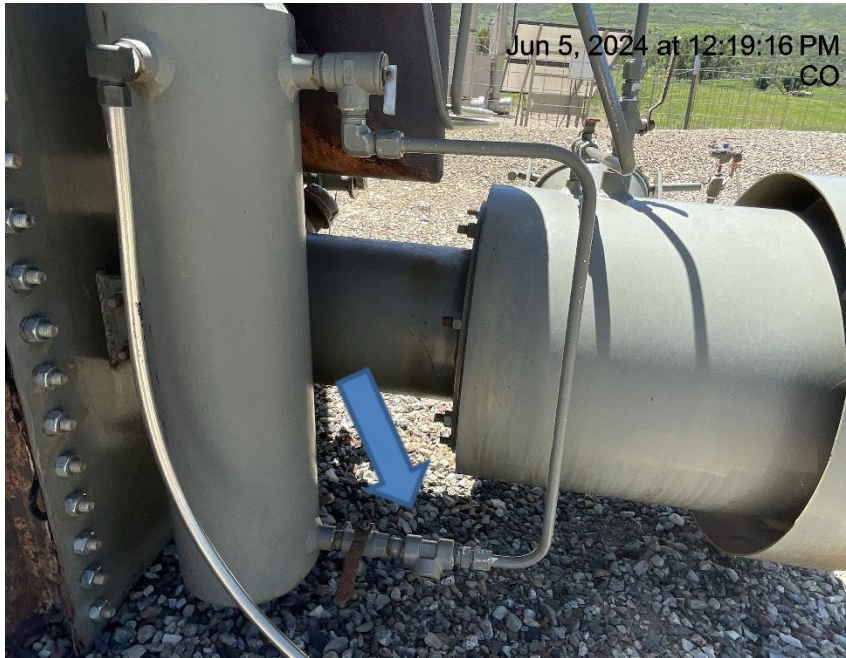
Photo # 9566 PRV vent line does not comply with CECMC pressure safety device rules
