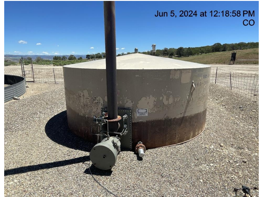
Photo # 9565 Tank lacks required labeling
