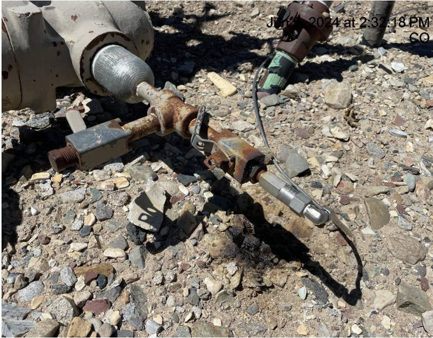
Photo # 9794 Staining near wellhead
