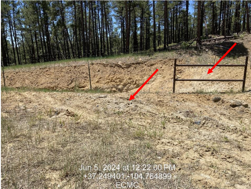
Photo 9 – Grey material noted around pit excavation
