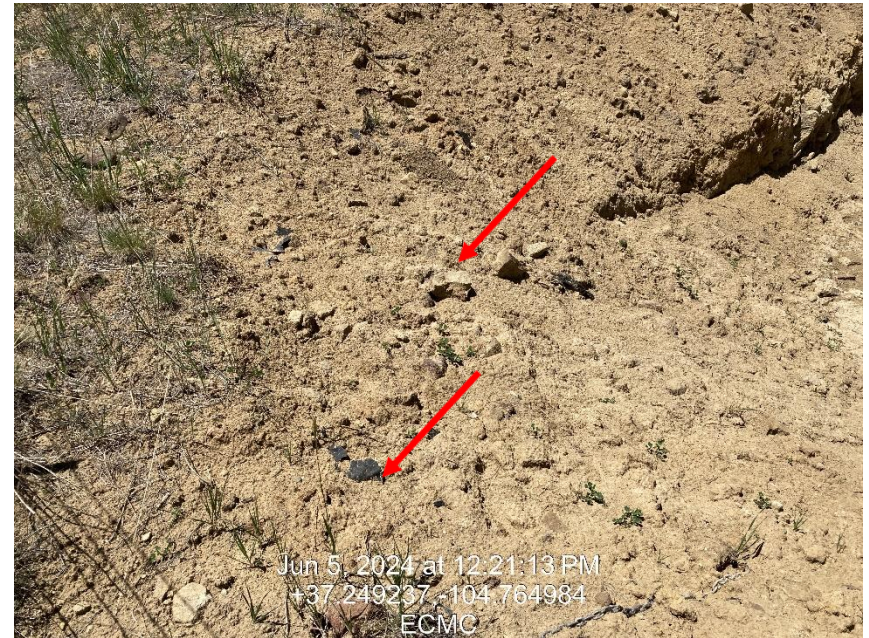
Photo 8 – Pieces of pit liner remain around top of pit excavation
