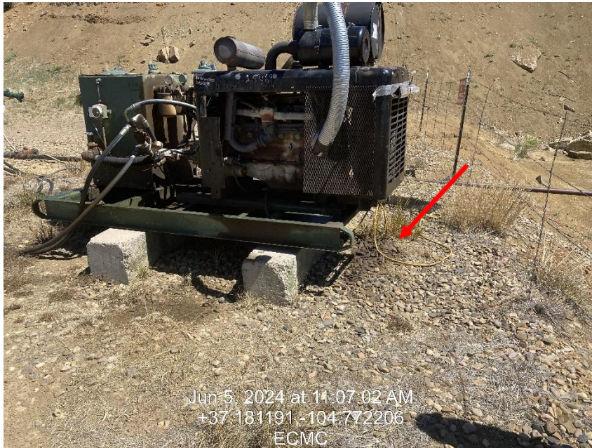
Photo 5 – Stained soils at engine skid
