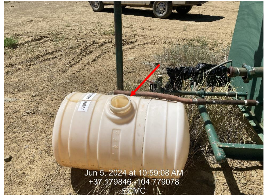
Photo 4 - Tank near Meter House missing cap
