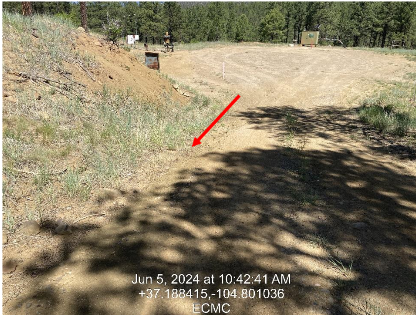
Photo 5 – Access road, stormwater is bypassing the culvert
