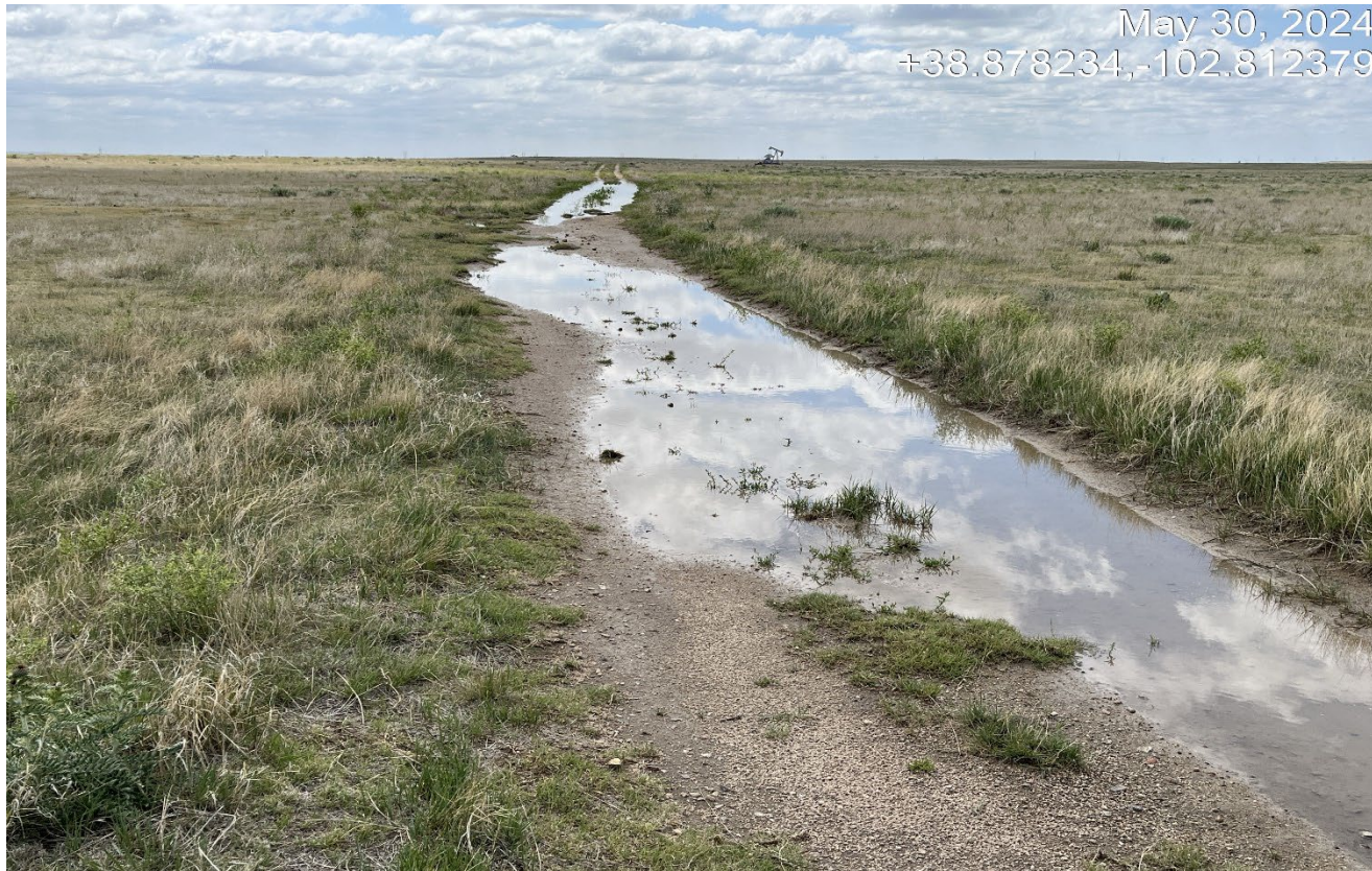
Photo 1. Facing southeast toward the access road. The access road was inaccessible due to water pooling on the road. The road needs to be built up with road base to allow proper stormwater drainage.
