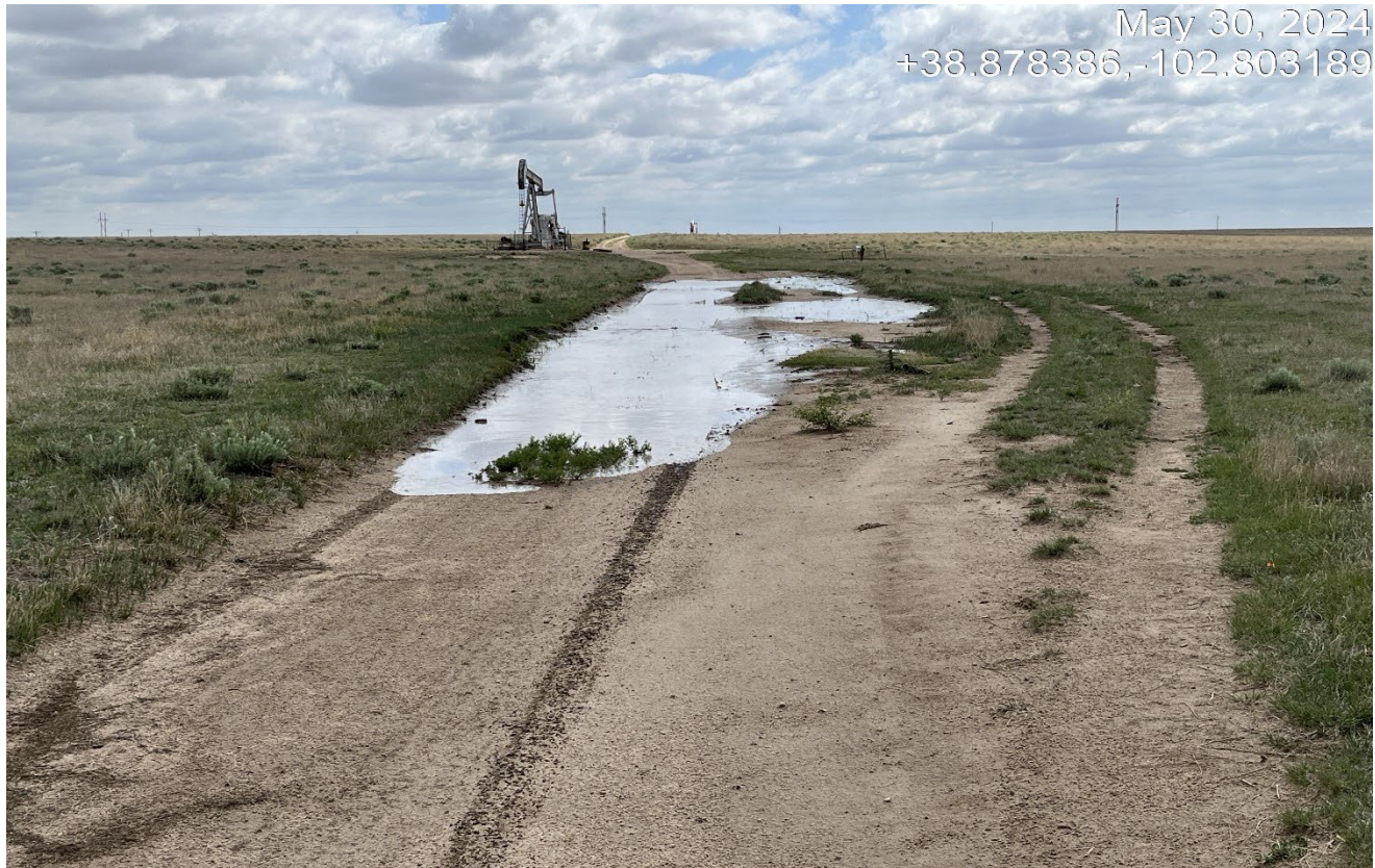
Photo 2. Facing east along the access road. Vehicles are causing unnecessary disturbance driving outside of the access road due to stormwater pooling on the road. The access road must be maintained and shall not drive outside of the access road boundary.
