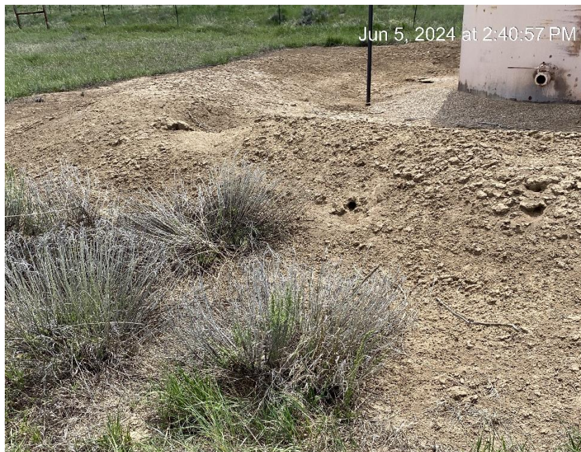
Berm undersize for size of tank
