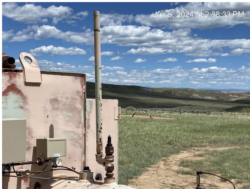
Relief riser missing rain protection
