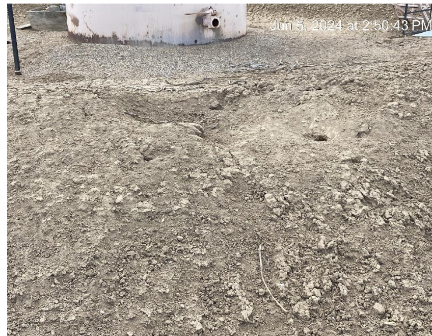
Berm not impervious to spilled fluids
