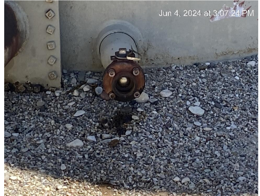
Open end tank valve. Oily waste. Stained soil.
