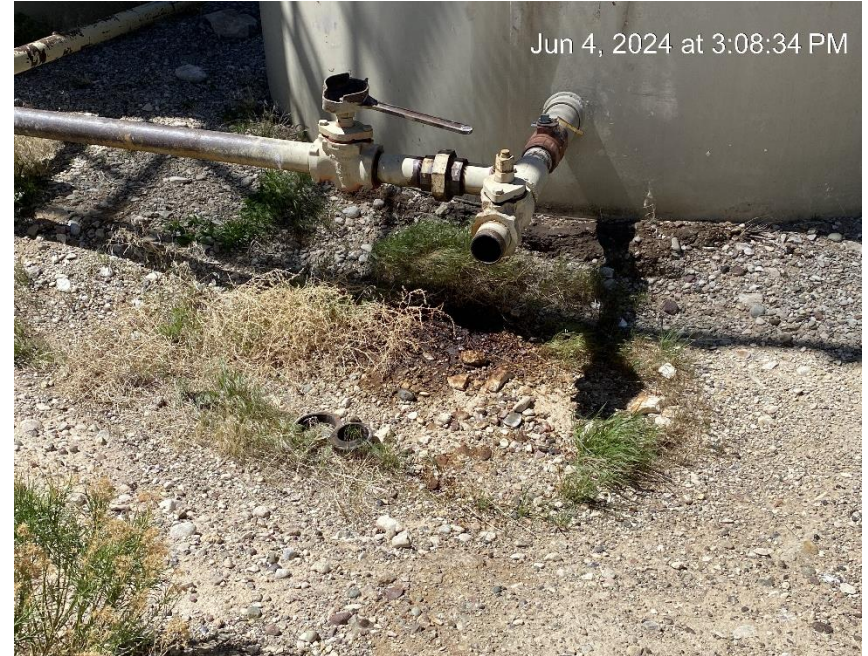
Oily waste. Open end tank valve
