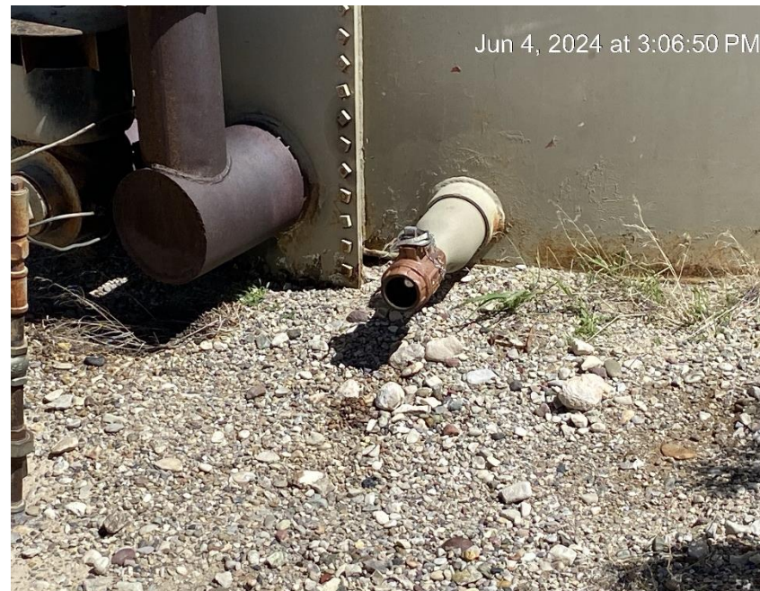
Open end tank valve. Stained soil.
