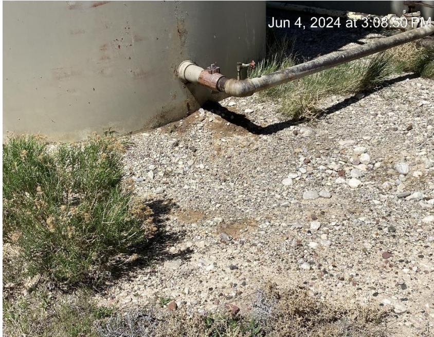
Oily waste. Open end tank valve.
