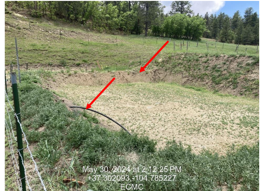
Photo 6 – Pit Facility ID 301143, Pit closure in process, flowline to pit remains in place. Material in pit bottom does not match pit photos from 10/31/2023
