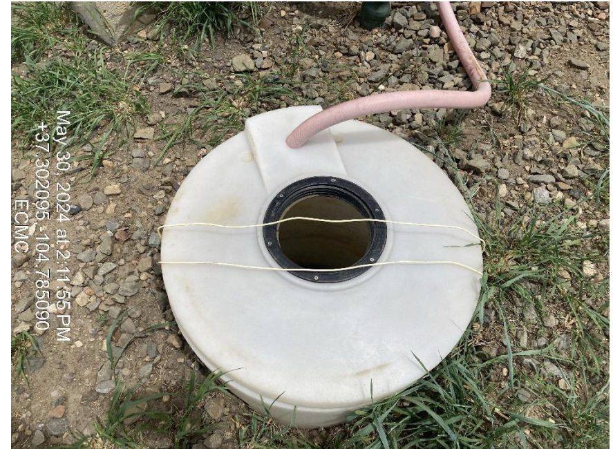
Photo 4 – Tank near meter house without cap
