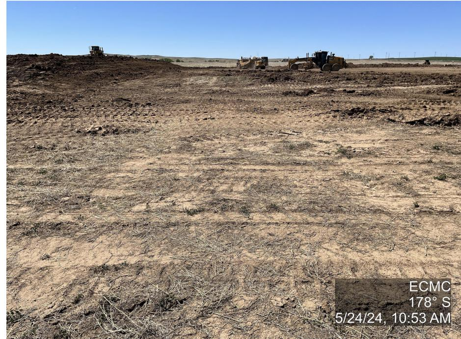
**Photo 5.** The photo was taken at the well location facing East. The photo illustrates topsoil removal in process as well as perimeter erosion control.
