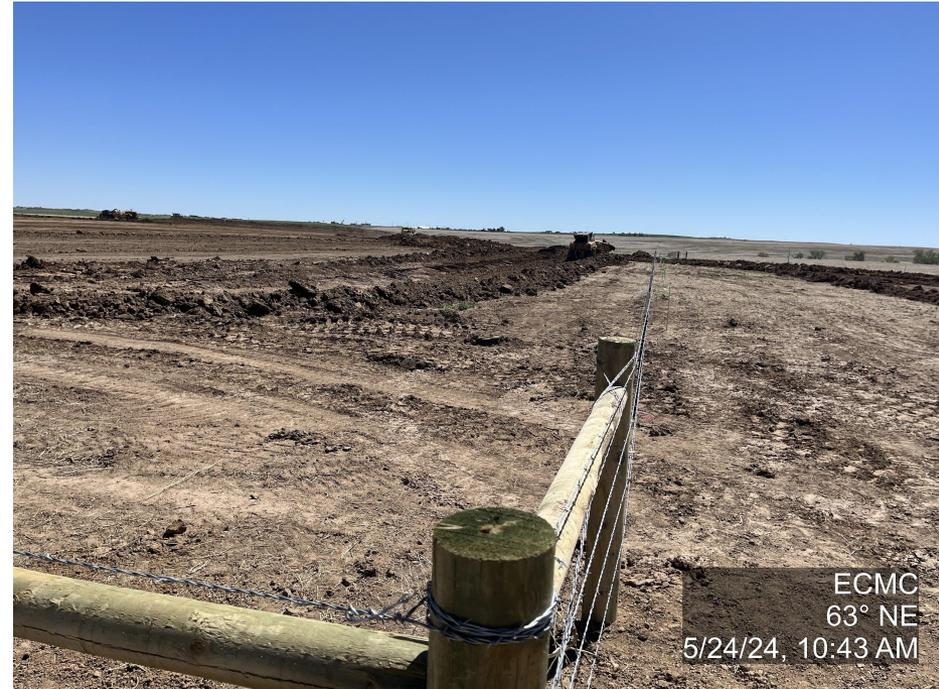
**Photo 3.** The photo was taken at the well location facing East. The photo illustrates the access road topsoil has been salvaged to either side and is still in the process of being stabilized.
