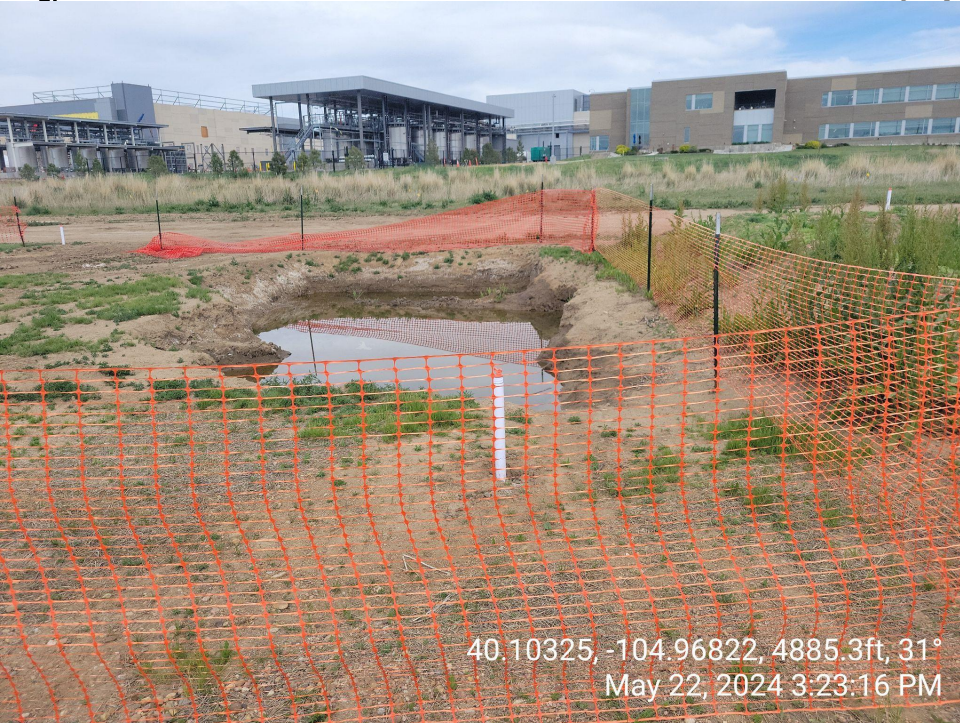
Johnson Battery Spill site. Excavation open and filled with water (groundwater)
