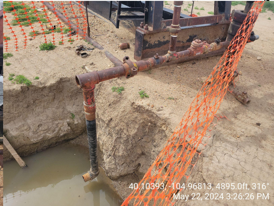
Johnson 1 Wellhead showing uncapped cut and removed flowlines, groundwater in excavation.
