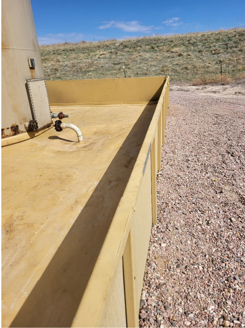
Photo Date 4/25/2024- Interior of containment with Liner in good shape.
