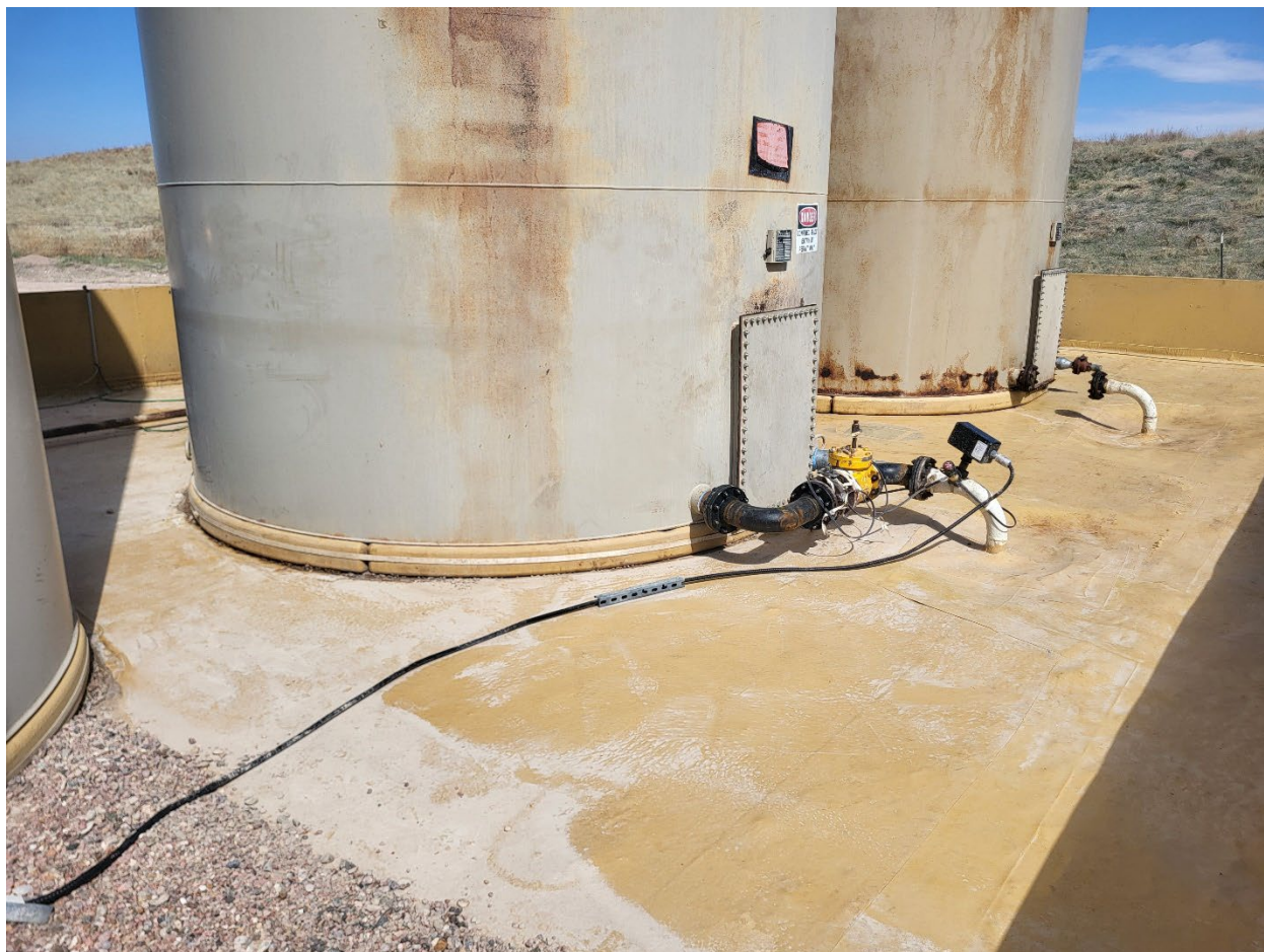
Photo Date 4/25/2024- Interior of containment with Liner in good shape in areas where release occurred.
