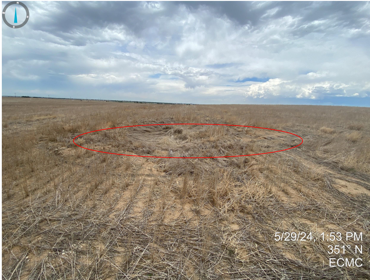
Photo 1. Facing north; the former wellhead area has subsided approximately 2-3' bsg. Additional reclamation activities are required to return the area to existing grade.
