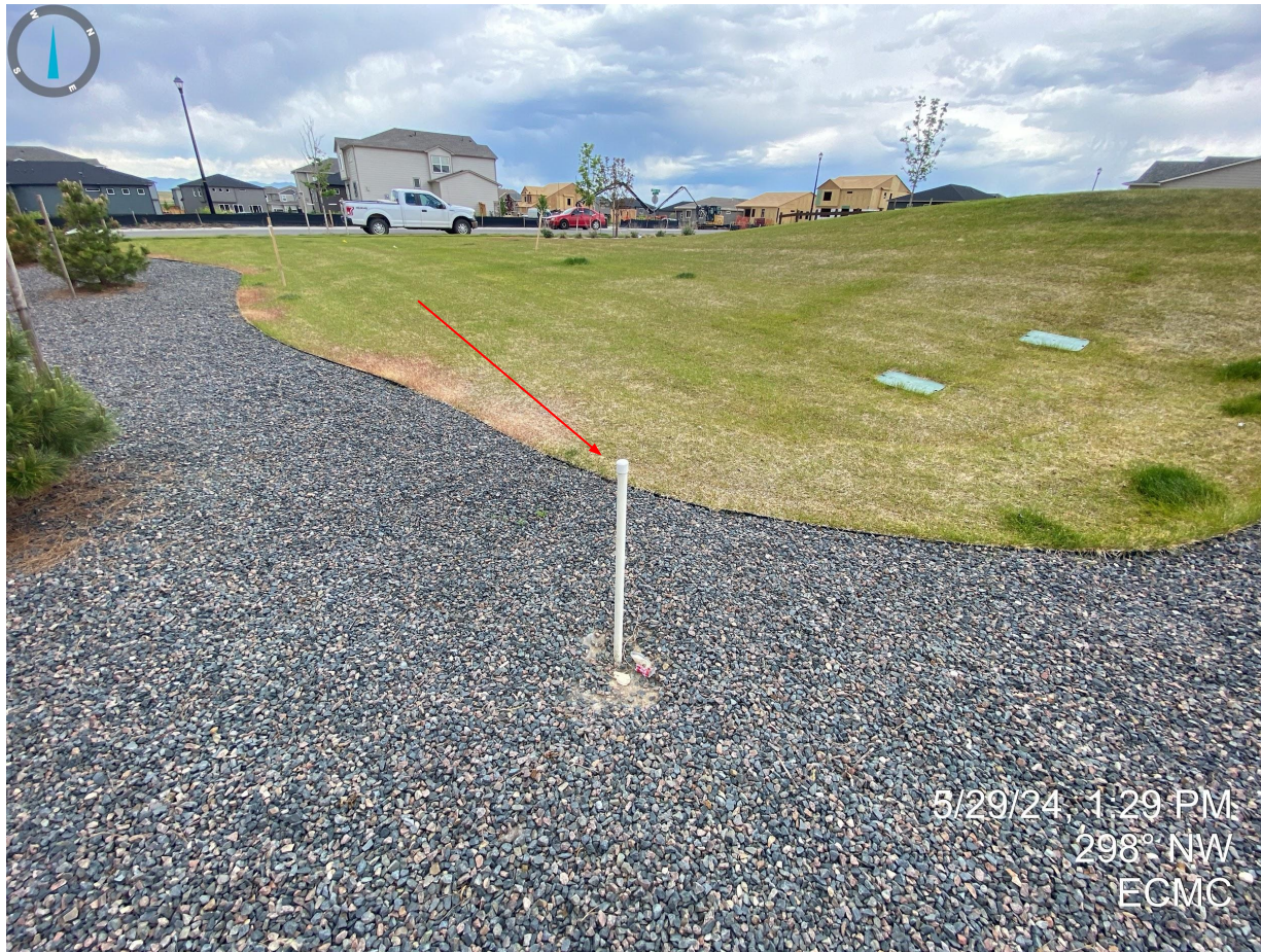
Photo 1. Apparent groundwater monitoring well remains on location and will need to be removed.
